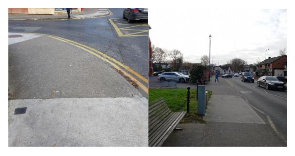
Desire lines, large radii junctions with undefined pedestrian routes close to Town Center Facilities and the lack of pavement contrast leave pedestrians, the visually impaired and mobility impaired isolated at primary crossing places.
