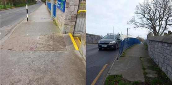
Incorrect use of tactile paving which is badly maintained, can lead to trips and falls.
