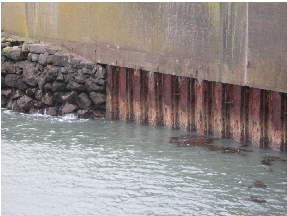
Fig B4 – Northeast Wing at Outpan No.1 – Typical Condition
