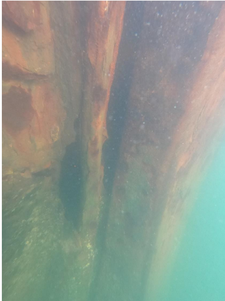
Fig B21 - Hole at MHWS level at corner with North – West Face. Outpan No. 111
