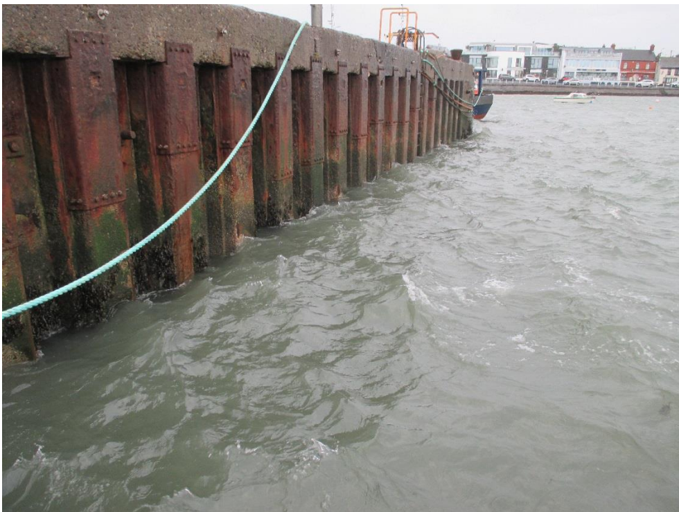
Fig B6 - East end of South Face
