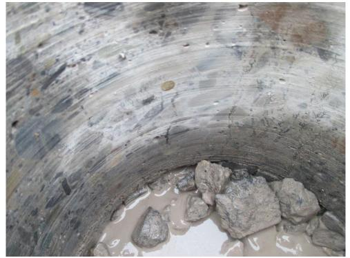
Fig 4.2.10 - Mesh Reinforcement visible within Hole No. 5
