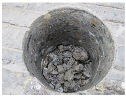
Fig 4.2.3 - Fill material within hole No. 2
