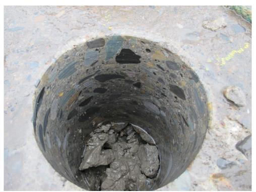
Fig 4.2.6 - Typical Slab Condition (Hole No. 3)
