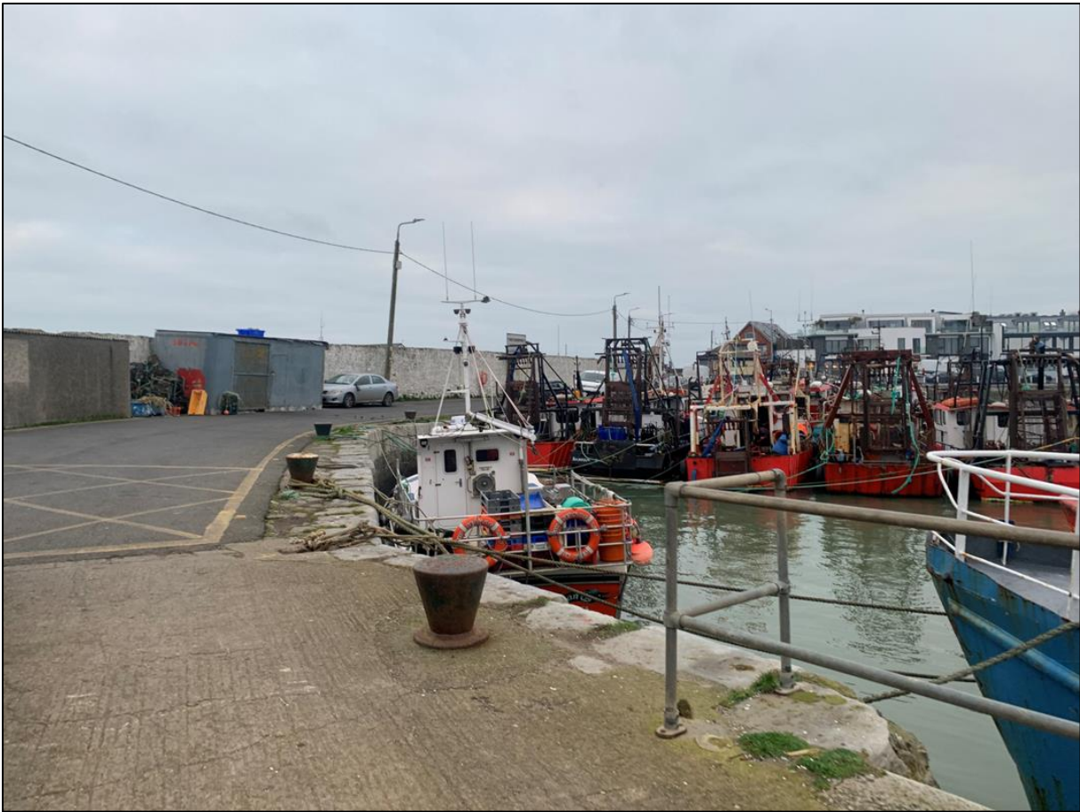
Figure 1-4: Additional views of Skerries Harbour and typical vessels that utilise berthing.
