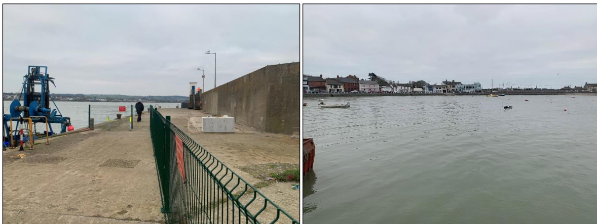
Figure 4-1: Additional views of the Skerries Harbour Pier and Skerries Harbour Bay.
