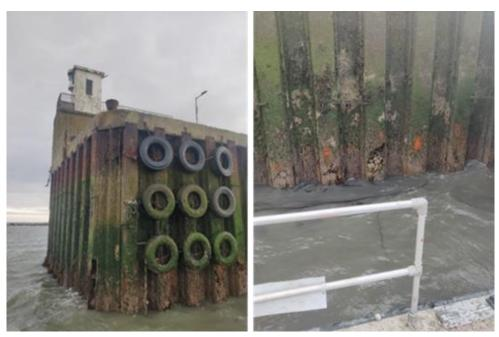
Figure 1-5: View of the Sheet pile pier and the extensive corrosion.
