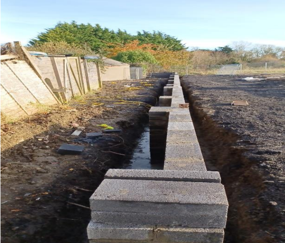
Laying of boundary wall foundations at Balgriffin cemetery
