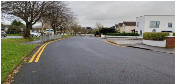
Double yellow lines added on Castleknock Avenue at the rear of the pedestrian crossing.
