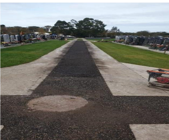
Balgriffin burial grounds ongoing hardcore works to assist funeral traffic vehicles and foot fall.
