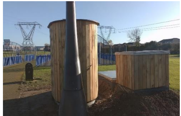
An Eco-toilet has now been installed this month in Tyrrelstown Park, beside the playground for use by all park-users.
