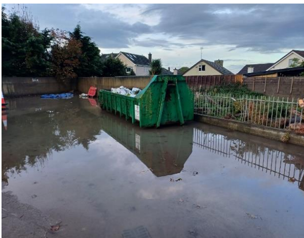
Drainage and flood relief works at St Fintan's burial grounds.
