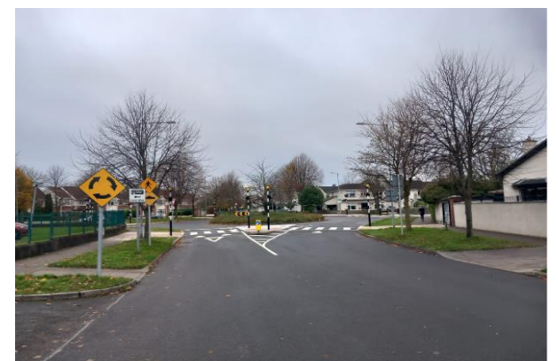
New four-arm raised zebra crossings on Carpenterstown Avenue/Laurel Lodge Road
