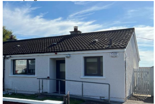
Post-works – Strandmill Estate, Portmarnock (external wall insulation, new windows and doors)
