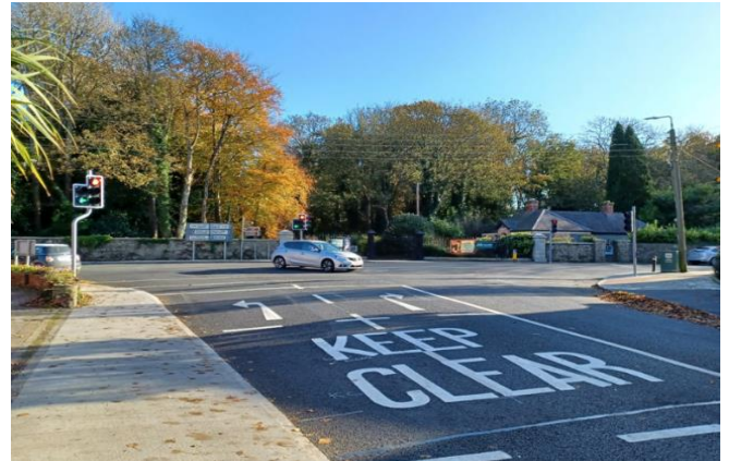
Examples of Road Marking and signage completed works in October 2023
