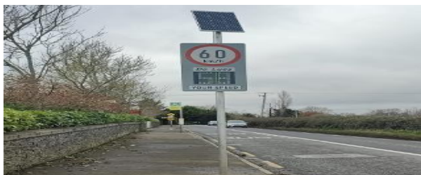
R125/Rathbeale Road Westbound at Kettles Country House Hotel – Traffic Calming - New Speed Reader Sign.
