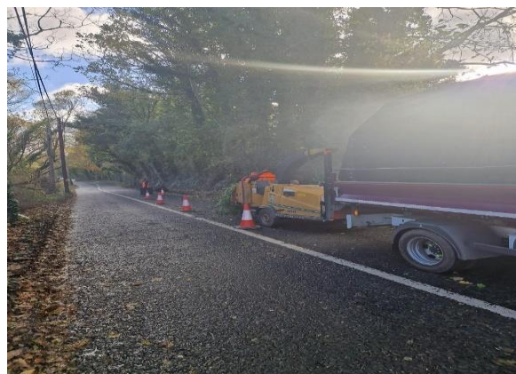
Fallen tree removal been carried out at River Road, Dublin 15
