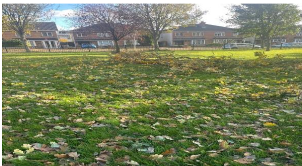
Clearing of trees at Littlepace Drive Open Space.
