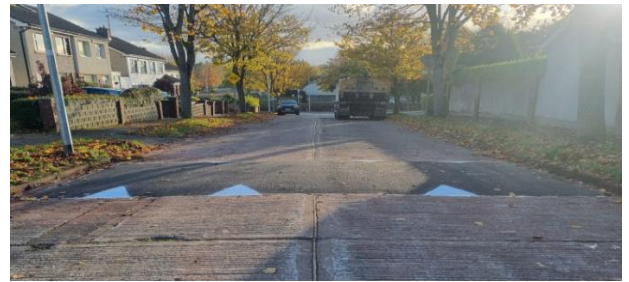
Hilltown Road, River Valley, Swords – Ramp Repair
