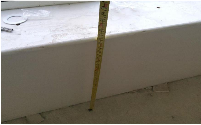
Checking window board height in a house in Carpenterstown (Part K)
