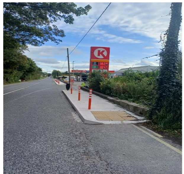
Kilshane – Concrete build out at Circle K
