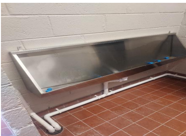
New urinal installed at St Fintans Burial
