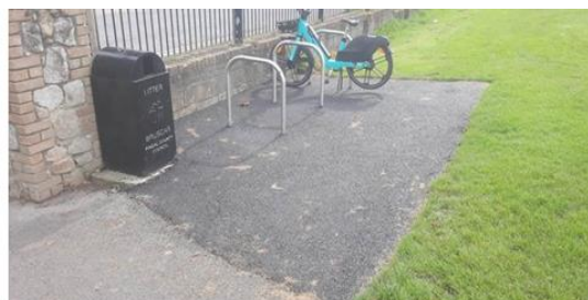
Recently installed Bicycle Stands at Dun Emer Avenue, Lusk, Co. Dublin
