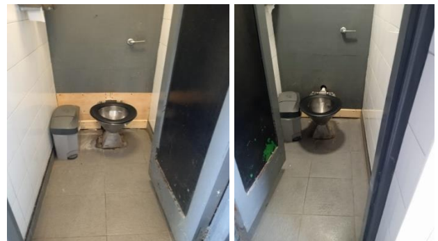
New woodwork access panels
