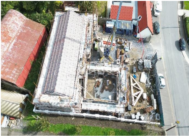
Fingal County Council - construction scheme at Monastery Court, Lusk – 5 dwellings
