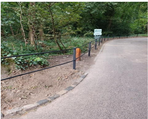
New Railing on McAlister Avenue, Malahide Demesne
