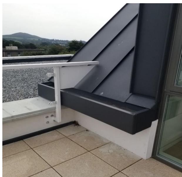
Checking Guard Railing on an apartment in Portmarnock
