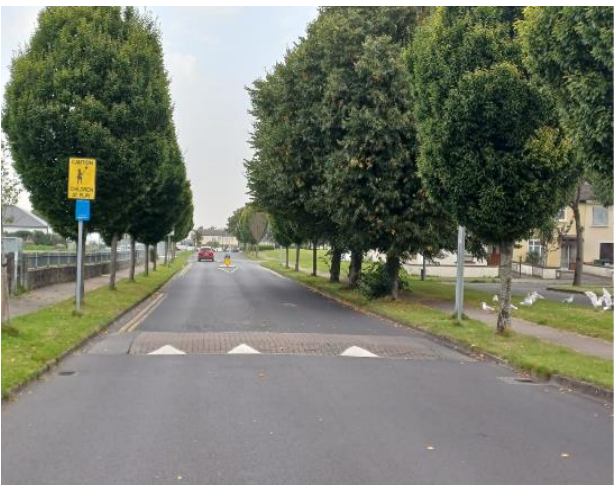
Lohunda Downs– Sharks teeth have been repainted onto existing ramps.
