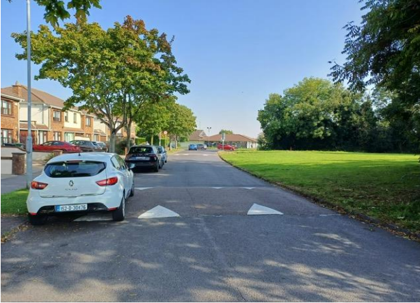
Oaktree Drive – Sharks teeth have been repainted onto existing ramps.
