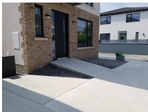
Checking access ramp in a house in Portmarnock.
