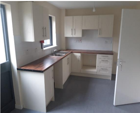
Kitchen/Bathroom refurbishments in Dublin 15
