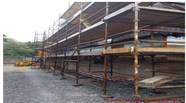
Fingal County Council – construction scheme at Bowden Court, Swords – 11 dwellings
