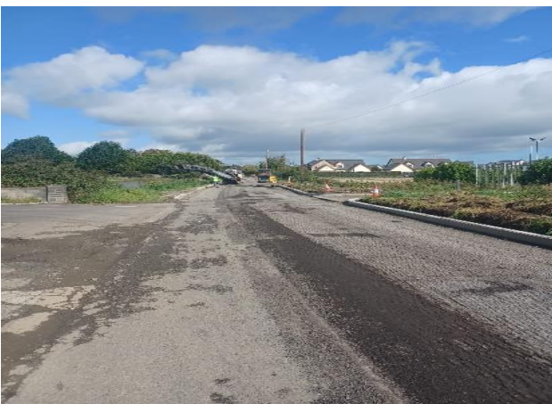
Road inlay works on Kinsealy Lane.
