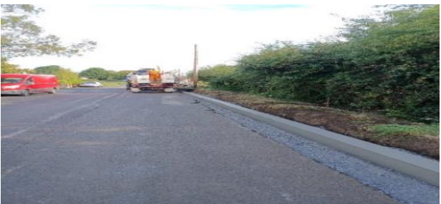
New kerbing being laid on Swords Road.
