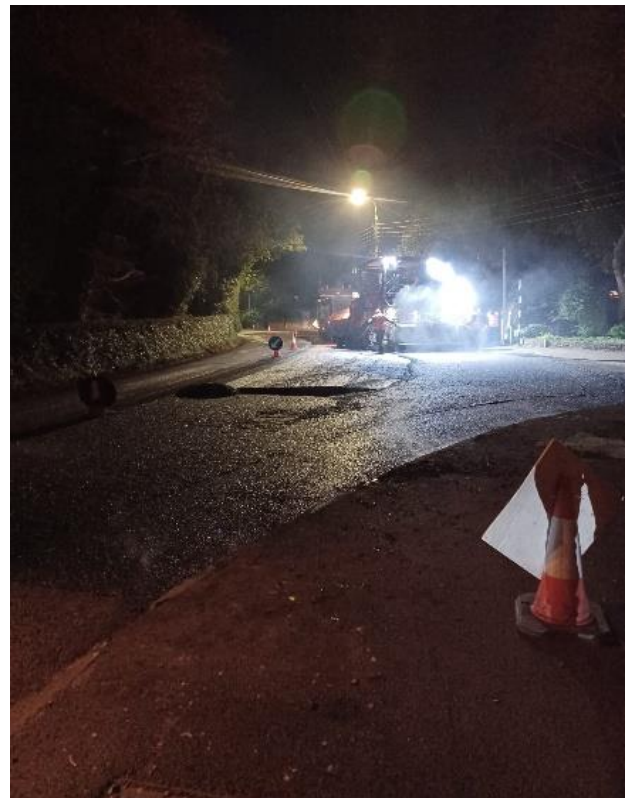
Night road works taking place on Swords Road.
