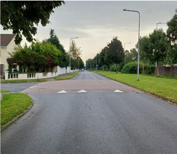
Lohunda Road – Sharks teeth have been repainted onto existing ramps.
