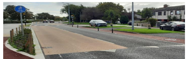
Anti-skid surfacing recently installed at front of schools
