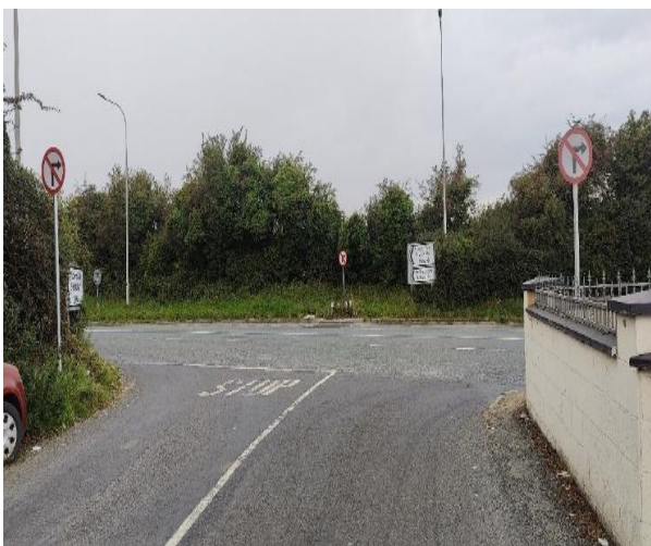
Kettles Lane at R132 - Further signage installed - Two 'No Right Turn' signs.
