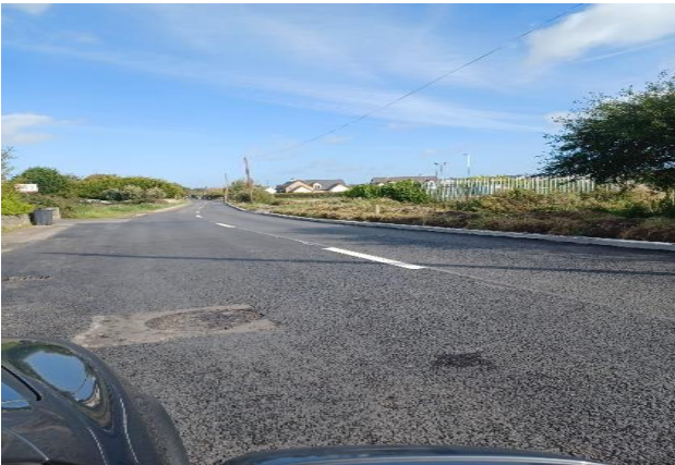
Kinsealy Lane prior to road inlay works
