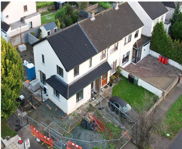
Fingal County Council - infill scheme at Clonsilla Road – 1 unit
