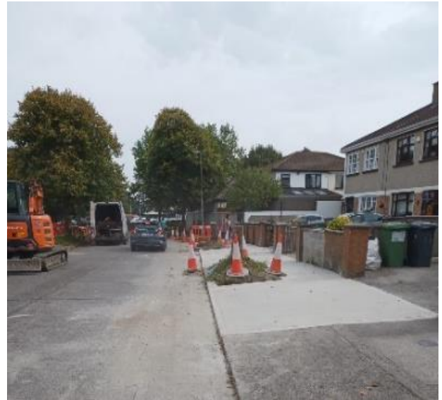
Ongoing path resurfacing works being carried out in the area.
