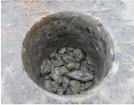
Figure 4-4: Fill Material Core Hole 1 (Norfolk Marine Ltd, 2021)
