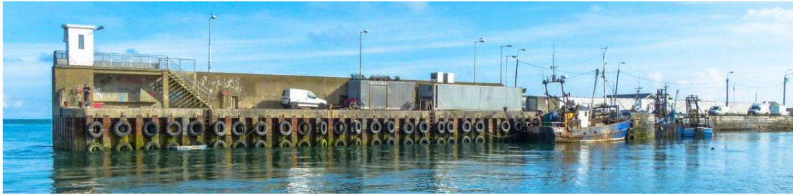
Figure 1-2: Skerries Harbour Pier Wall (eOcenic, 2023)
