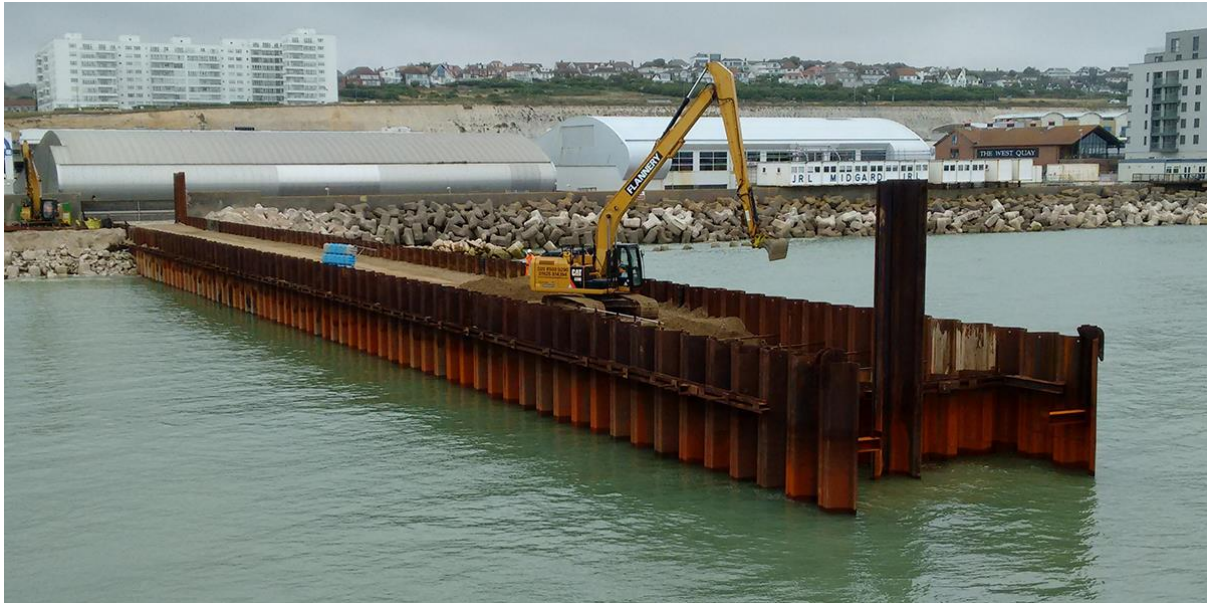
Figure 8-6: Example of Sheet pile Pier Under Construction (source https://shorturl.at/azS27 )
