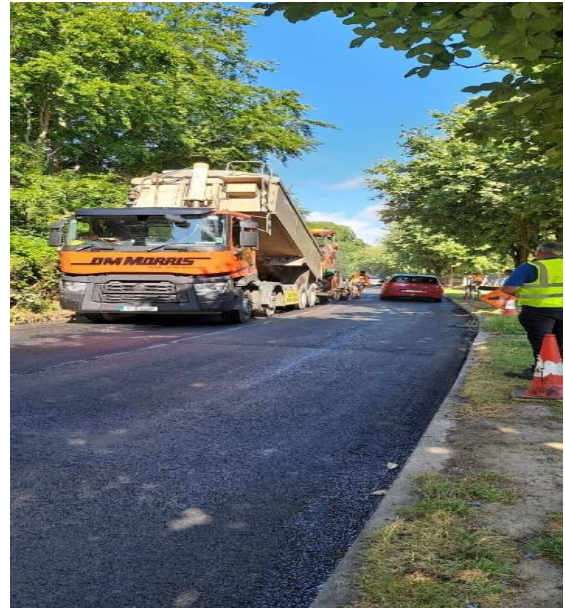
Donabate Turvey Avenue Road inlay works
