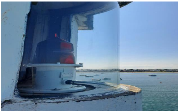
Replacement of Skerries Lighthouse window from plastic to glass
