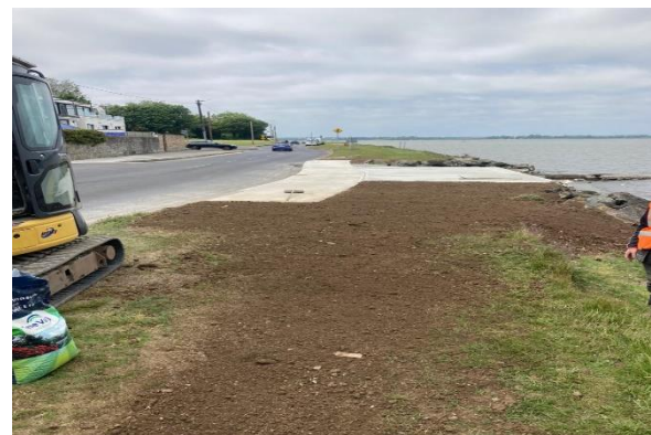
Path repaired and jetty Cave Strand, Malahide. Work by contractors
