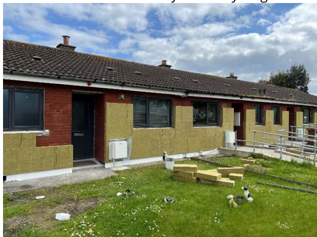
External Wall Insulation underway in Strandmill Estate, Portmarnock.
