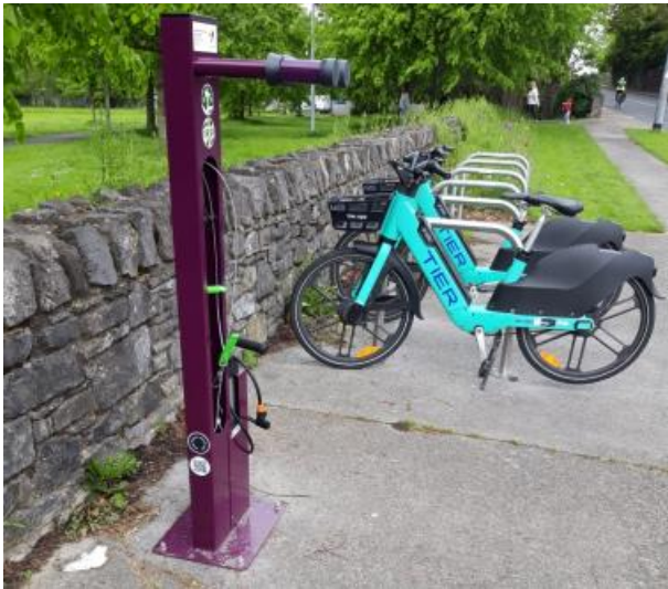
Recently installed bike repair station
