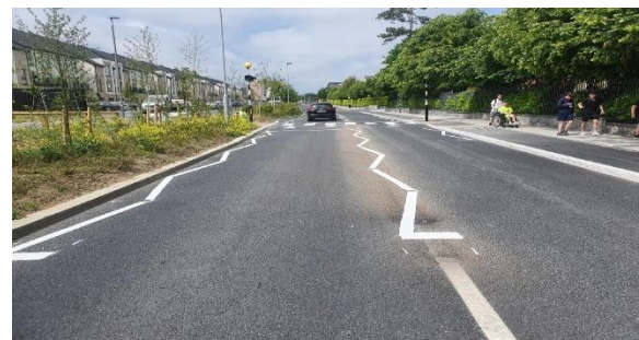
Pedestrian crossing installed on station Rd.
