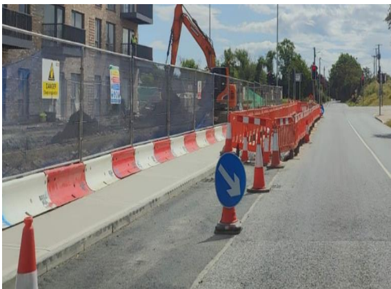
New Road junction with R126 Donabate Distributor Road
