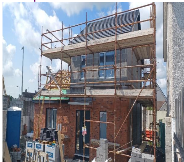
Fingal County Council - infill scheme at Sheepmoor Avenue - 1 unit
