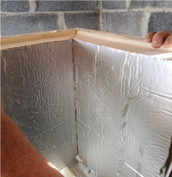
Checking Insulation in a housing development in Lusk.
