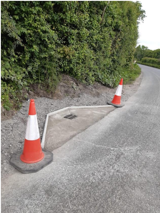
New Gully installed by Balbriggan Roads Crew at area previously prone to flooding in Walshestown.
