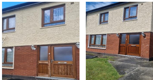
Before and after painting pictures taken in Sheephill Estate, Blanchardstown
