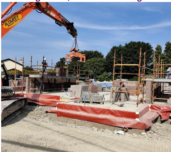
Fingal County Council - construction scheme at Ballough Place, Lusk - 10 dwellings
