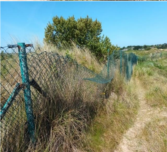
Repair to dune fencing at Portmarnock Beach
