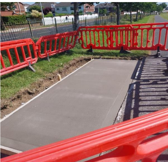
Concrete footpath repair works by internal Operations crew at Pine Grove, Swords
