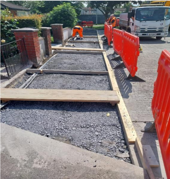
Concrete footpath repair works by internal Operations crew at Pine Grove, Swords
