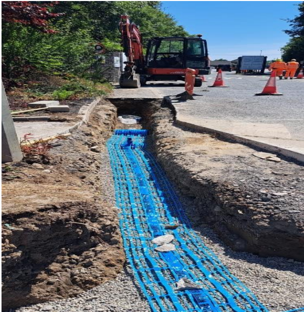
Water main installation works for Estuary Recycling Centre, Swords
