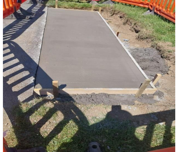
Installation of Park Bench bases at Brackenstown Road, Swords
