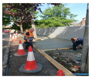
Depot Works: Roads crew replacing tree damaged footpaths at Glencarraig, Offington
