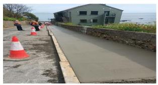
Howth Malahide Operations designed and widened footpath the full length of Balscadden Road Howth. The crew poured approx. 250m length of concrete paths.
