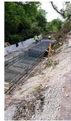
Brackenstown Road Subsidence works. Gabion baskets being filled for road re- enforcement
