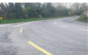
Ballymadun- New lining to improve road safety on the approach of the bend. New warning signage installation in progress.
