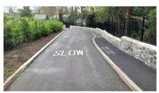
Before and after photos of road widening and new footpath in Shackelton's leading to gardens area Improvement works to widen at the bend in road for vehicles, also a new stone wall and railings on right hand side of road with designated footpath and bollards for pedestrian walkway
