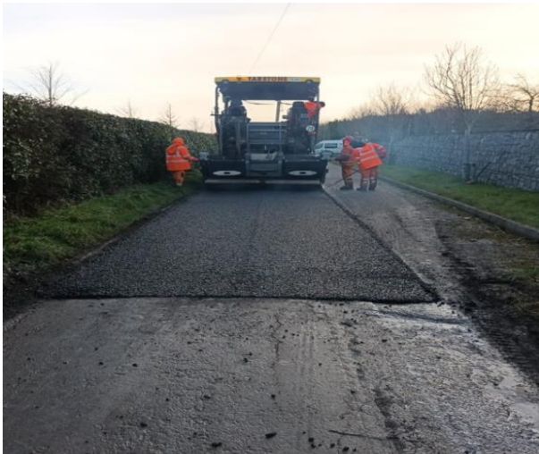
Asphalt paver in operation - Drisgoue Road
