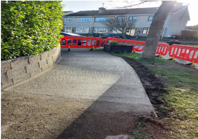
Fresh concrete outside 63 Fancourt Heights
