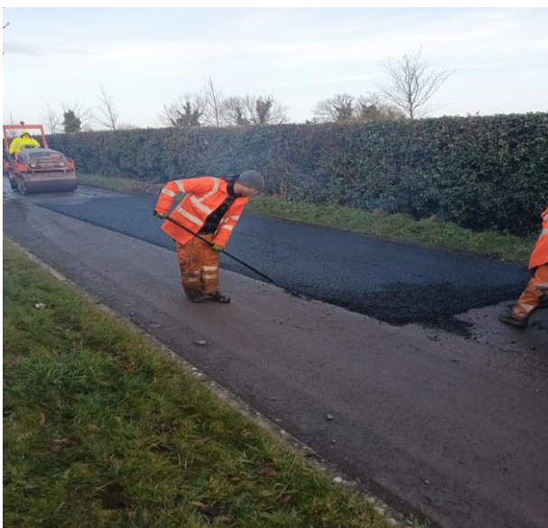
Placement and compaction of tarmac during road reinstatement – Raheny Lane, Lusk
