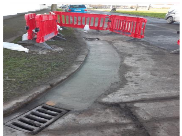
Repair gully connection Newtown Park, Skerries
