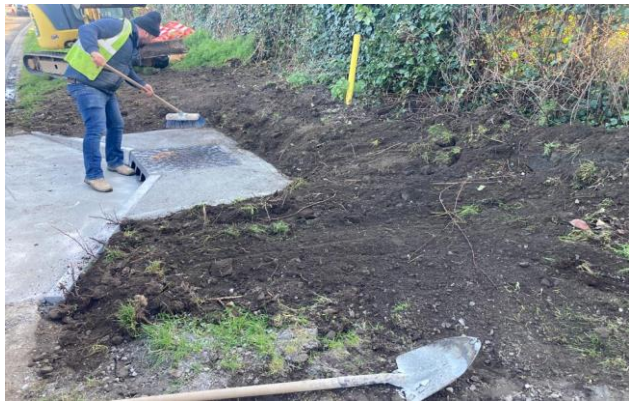
Recessed side inlet kerbed manhole
