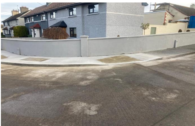
Designated pedestrian crossing points with tactile pavement slabs
