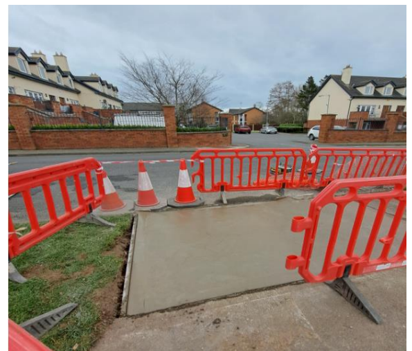
Donabate, Beaverstown Orchard, footpath dishing under construction.
