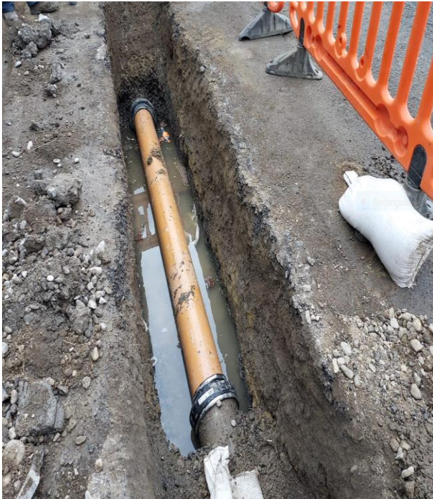
After - repaired section with uPVC and collars
