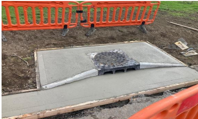
Recessed side inlet kerbed manhole
