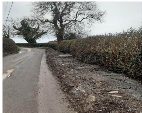
Backfill and completion of works
