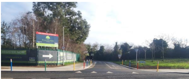
Raheny Close junction upgrade
