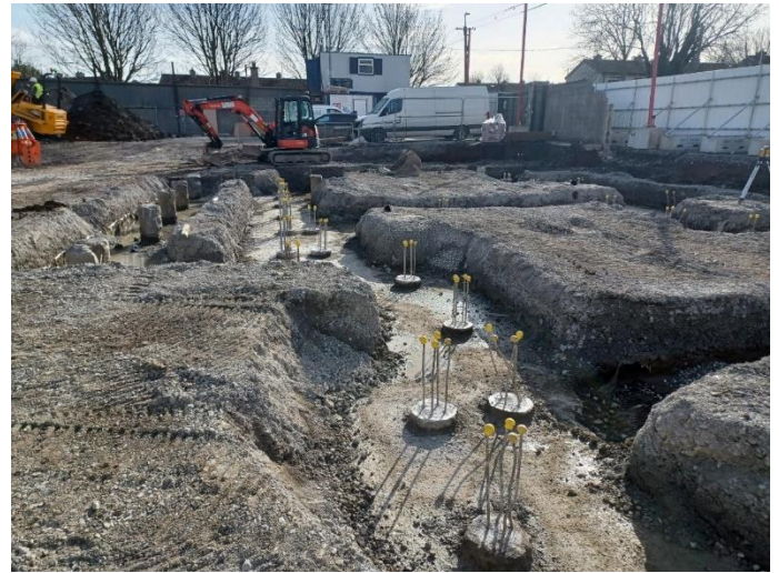
Fingal County Council infill scheme at Clonsilla Road, Dublin 15
