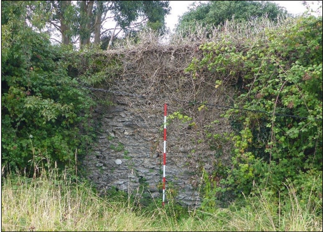
Plate 11 Boundary to walled garden with rubble-stone facing intact
