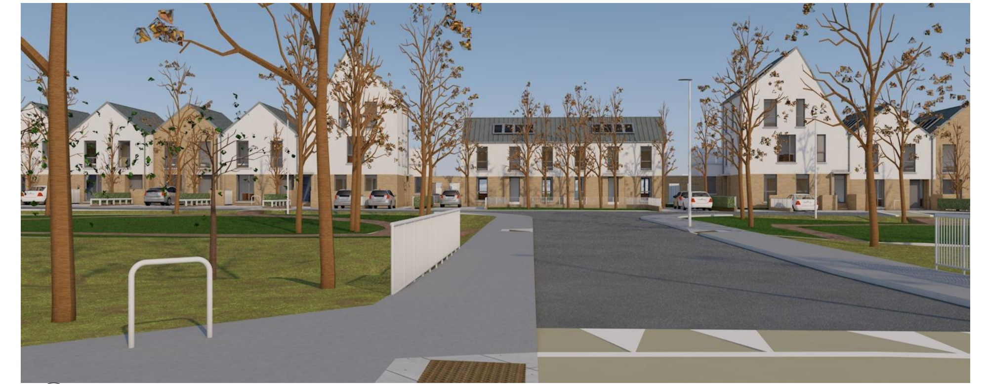
06 400 NORTH SIDE FROM MAIN ROAD
