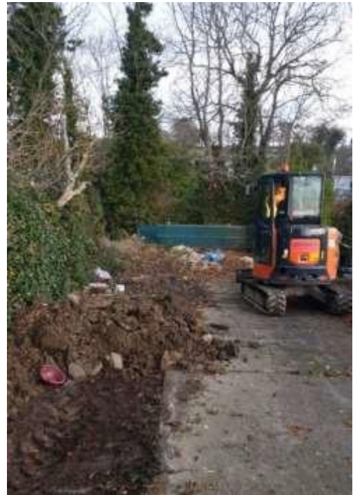
Works ongoing on winter hedge and bank clearance.
