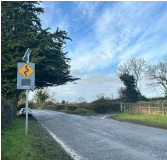
L1080 Hollywood- VAS installed to warn drivers and provide speed feedback
