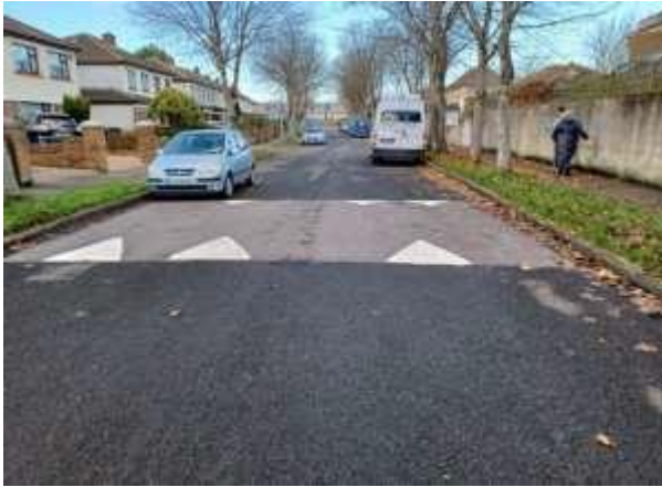
Sharks Teeth renewed on all nine Traffic calming ramps along Seabury Crescent
