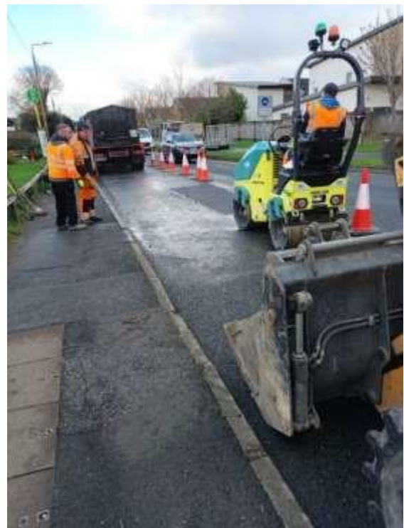
Roads Crew patching Swords Malahide Road
