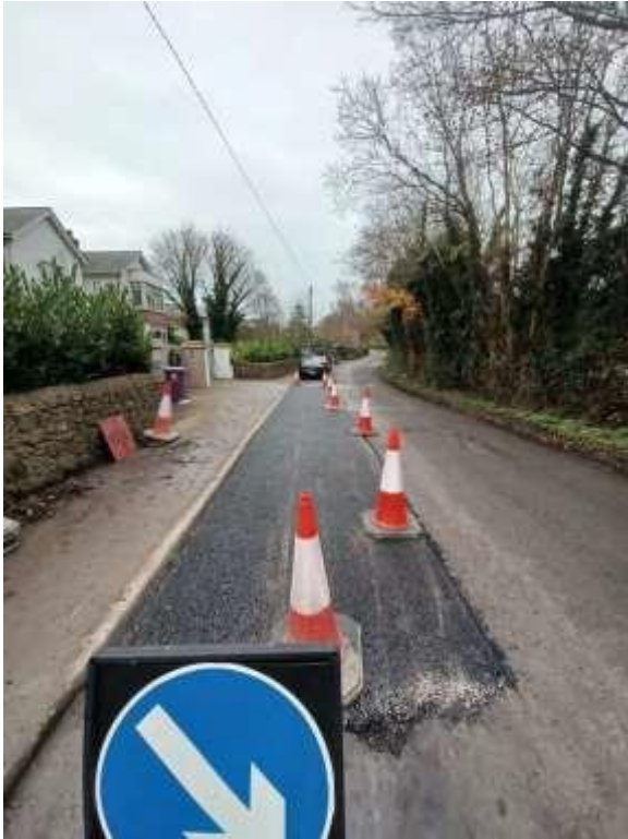
Roads Crew patching Streamstown Lane
