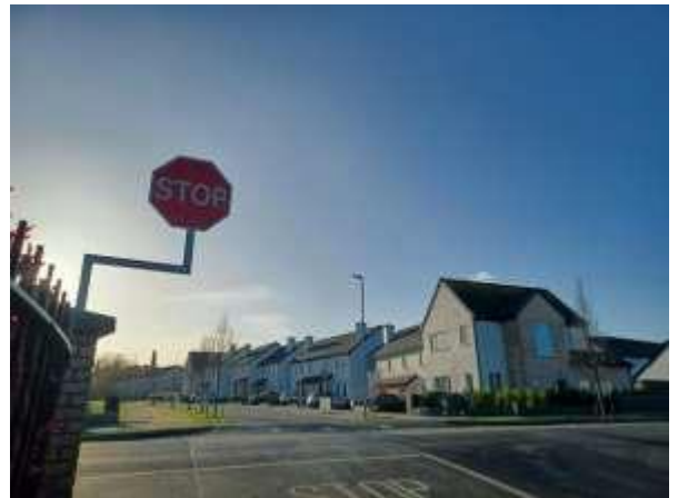
New 'STOP' Sign on cranked pole at junction of Kinsealy Lane and Chapel Road
