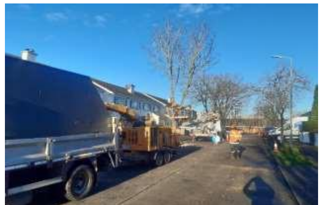
Clearing green waste in Dromheath Drive
