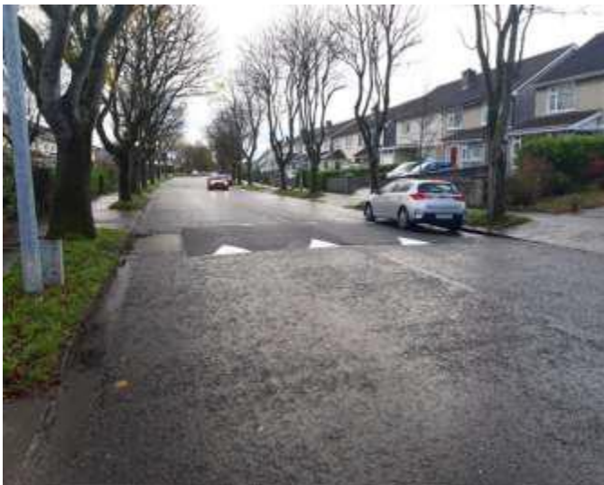
Newly repaired ramp on Roselawn Road
