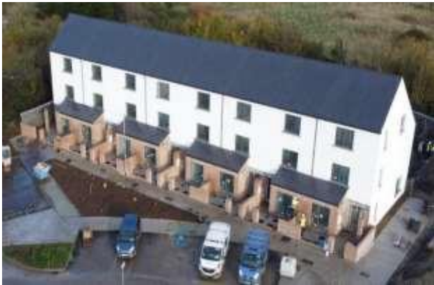
Fingal County Council construction scheme at Wellview, D15 – 20 units being built
