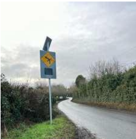
Oldtown- VAS installed approaching the junction between R122 and R129.
