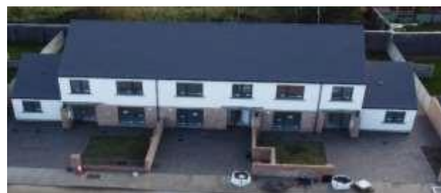
Fingal County Council construction scheme at Cappagh, Dublin11 - 69 dwellings
