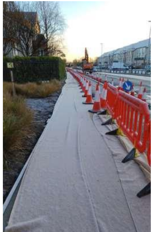
Cycle Lane Concrete Poured
