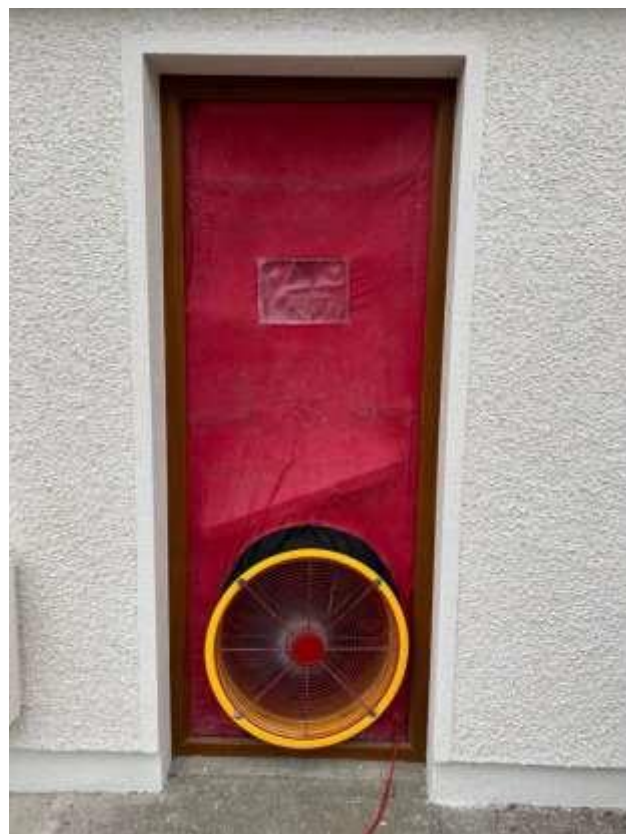
Air tightness test in progress
