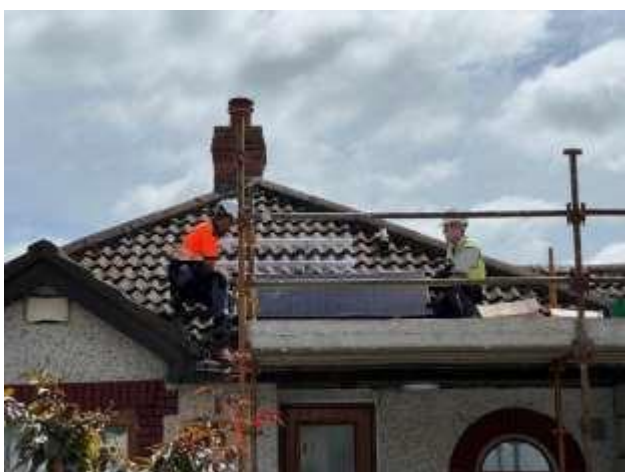
Fitting solar panels in Jugback Estate, Swords
