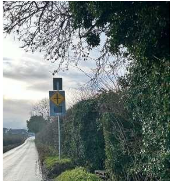
Garristown- VAS Installed at L1006 southbound towards Garristown Main Street
