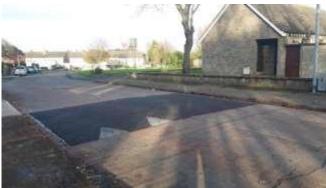
Swords – Glasmore Park – Ramp replacement
