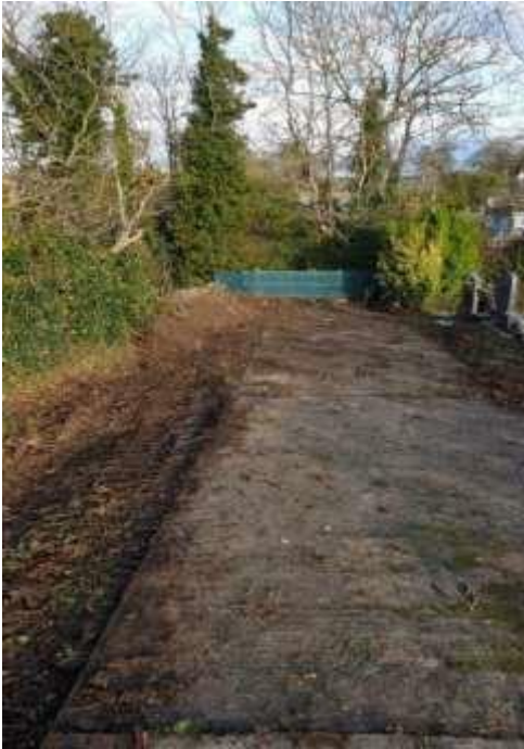
Completed view following works in Balgriffin Cemetery
