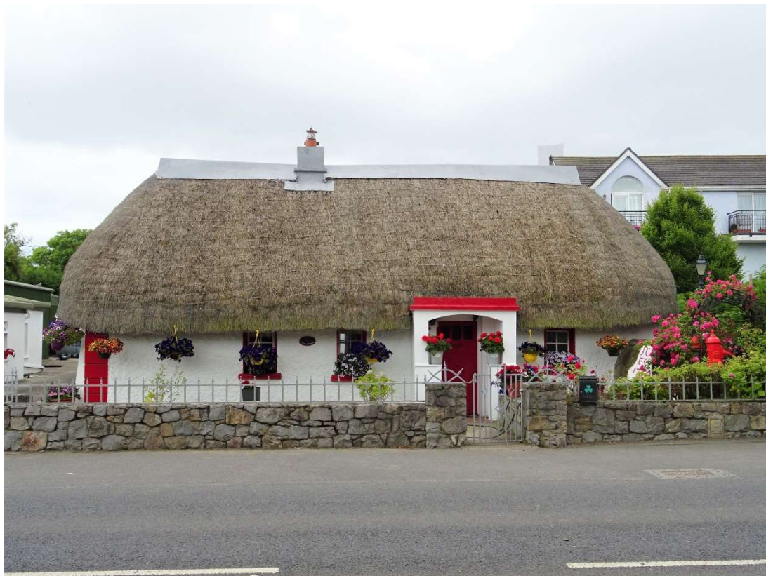
Clay Cottage, Dublin Road, Lusk which has a steel ridge
