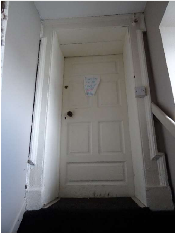
Left: A lugged and kneed architrave from the mid-18 th century which is an unusual feature within a thatched house.
