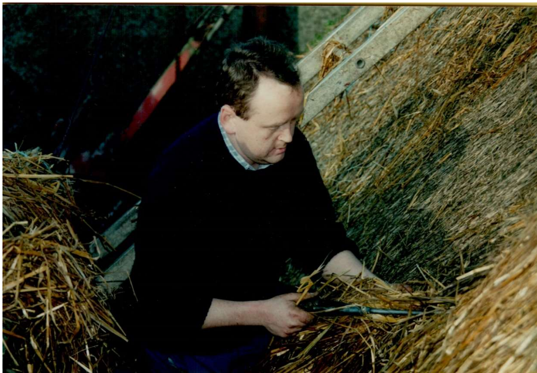
A photograph of Martin Fanning, son of Charlie, slice thatching a roof in Fingal. Courtesy of Martin Fanning
