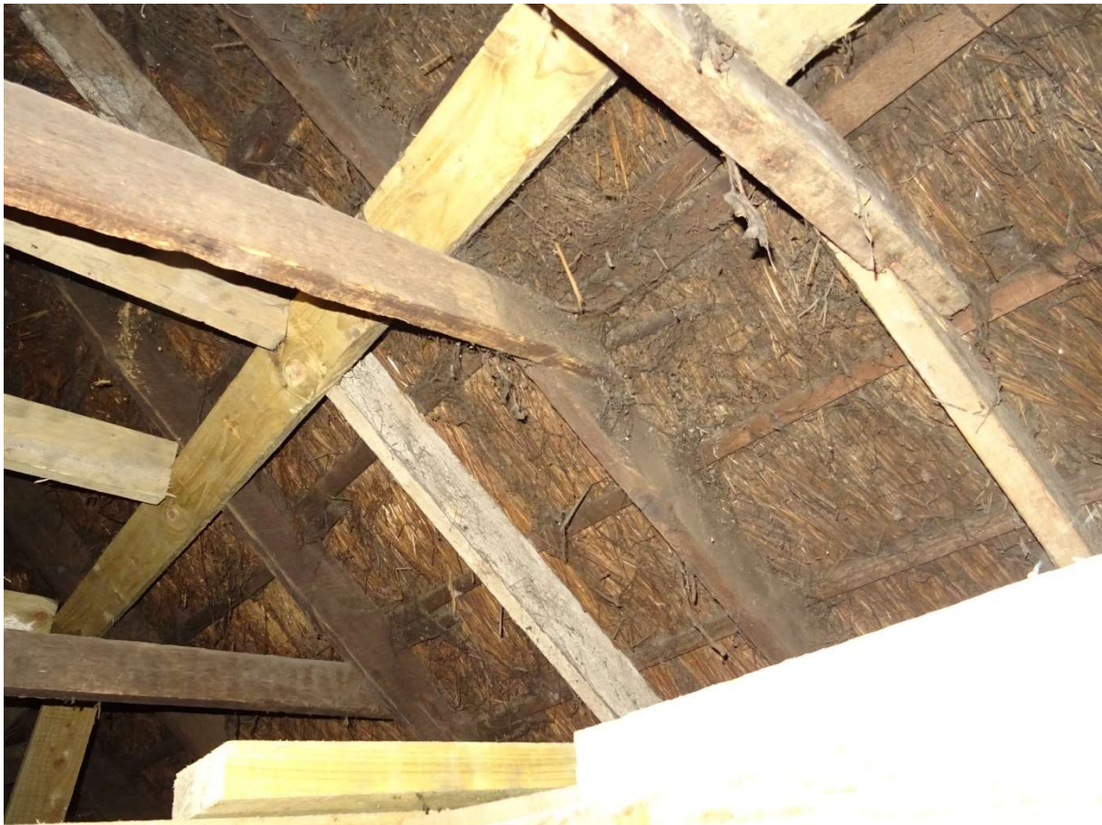
Roofing timbers with additional supports to Clay Cottage, Dublin Road, Lusk
