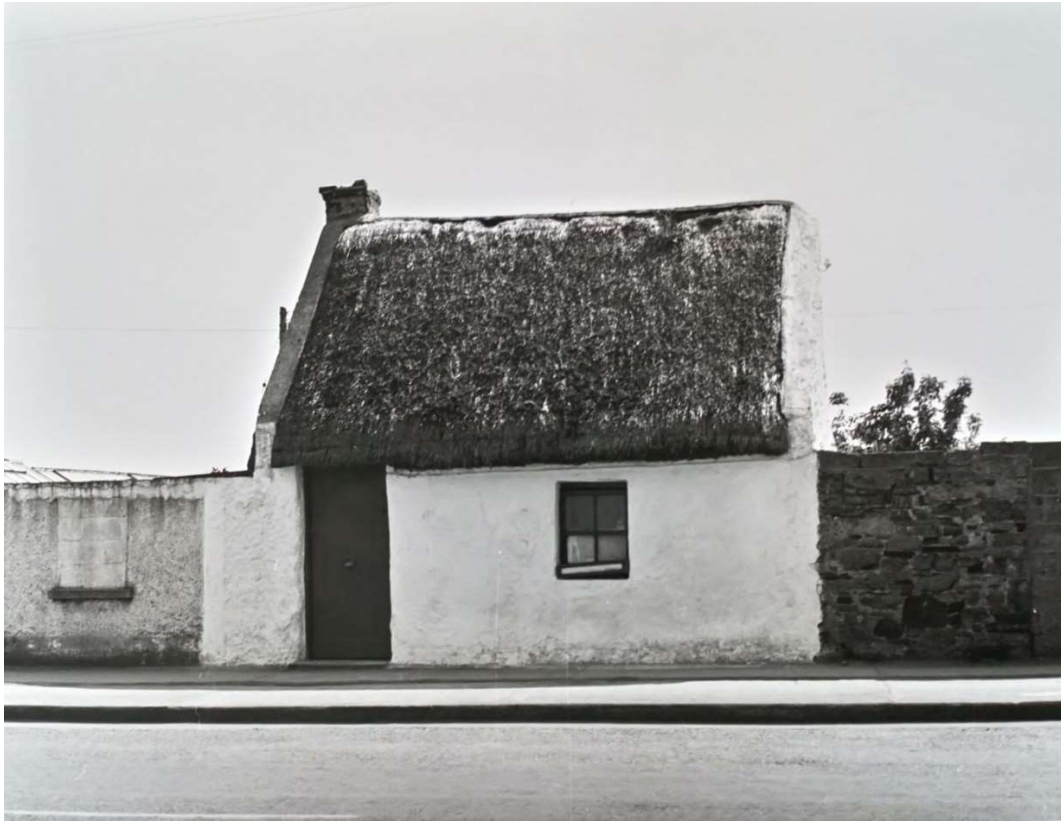
A clay ridge to Johnny Donnelly's house at Lower Main Street, Rush, now demolished. Photograph taken by Kit Sheridan c.1975, courtesy of Niall Gosson
