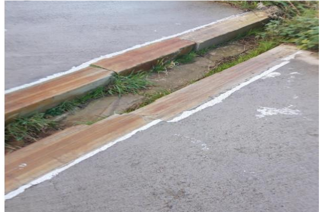
Before: Howth Cliff Walk Works
