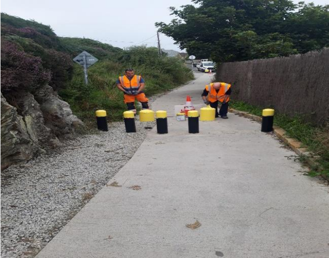
Works to improve visibility of obstacles at Howth
