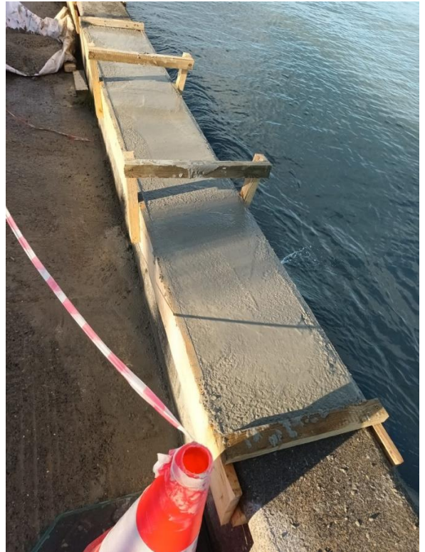
Capping works with shuttering
