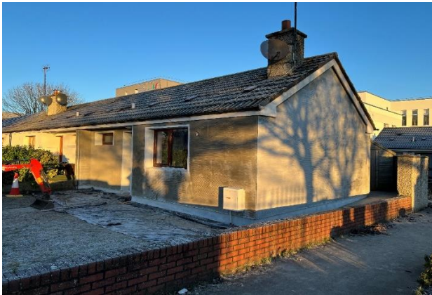
External insulation underway in St. Paul's, Balbriggan.
