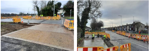
Figures 1: Junction upgrade works at Brackenstown Road and St. Cronan's junction
