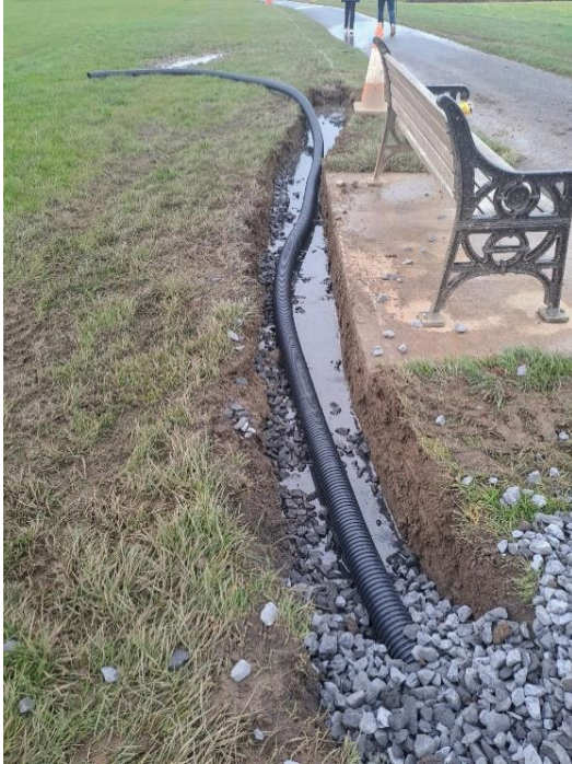
Paddy's Hill Drainage Works
