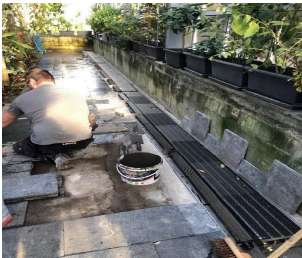
Ongoing work showing underground heating before grilles are in place
