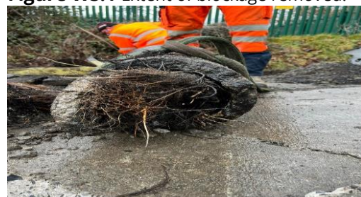
Figure WS.1 Extent of blockage removed.
