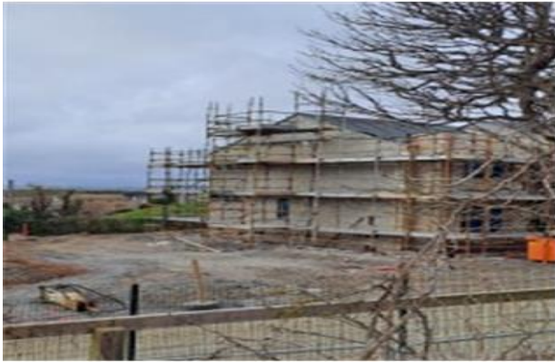
Part V Units under construction at Seamount, Malahide, Co Dublin
