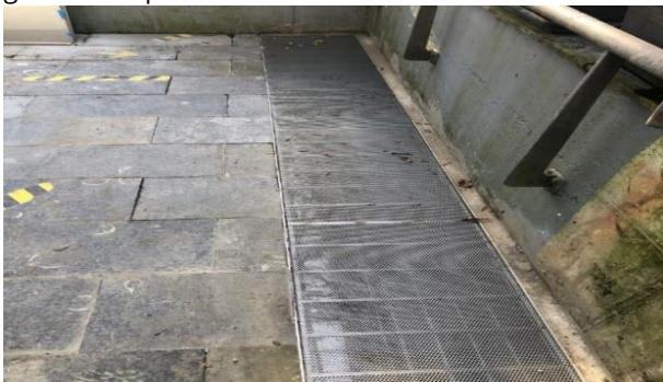
Underground heating trench complete with new grilles in the Butterfly House
