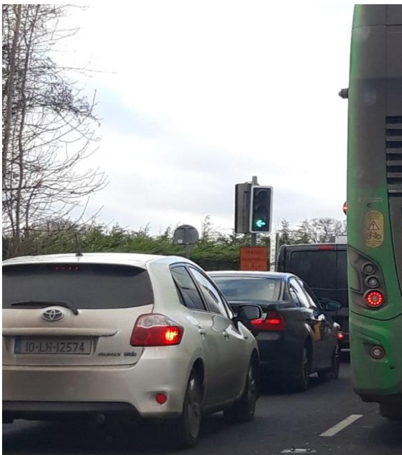
A left turn only filter light has been added to the off-ramp on Junction 4 on the M3
