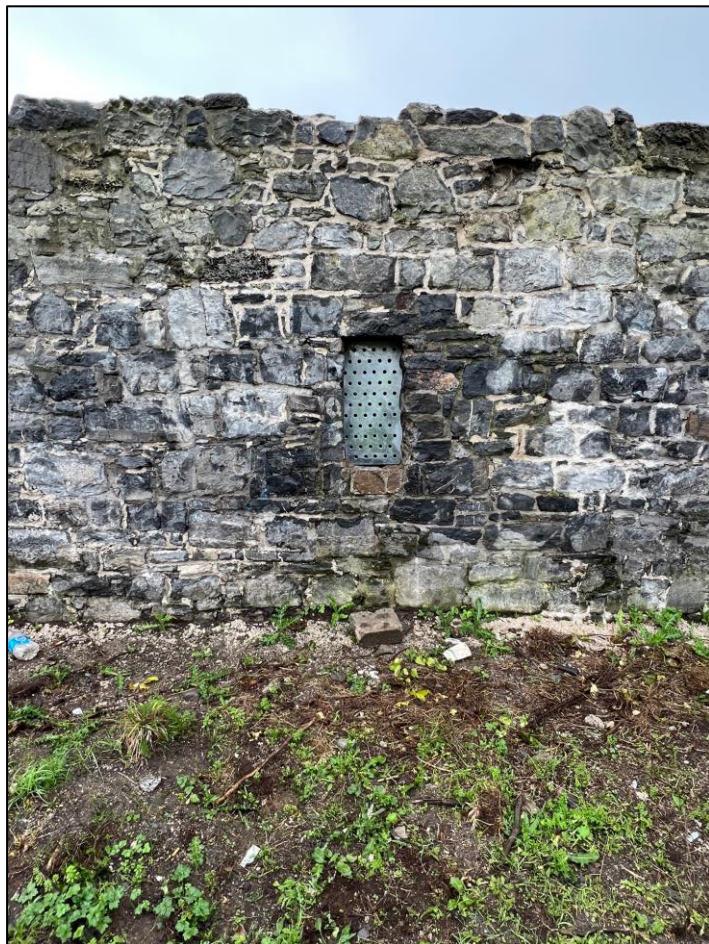
Plate 11 Eastern elevation post graffiti removal, with secured ope, facing west
