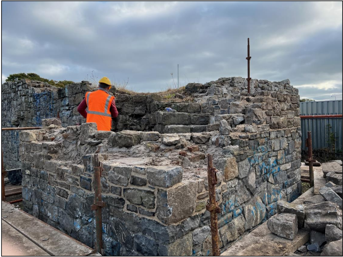
Plate 7 Rebuilding of corner tower, facing southeast
