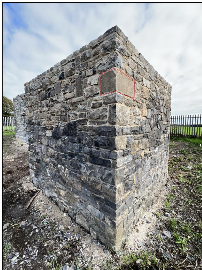
Plate 14 Partially rebuilt corner tower, with re-used quoin stone highlighted in red, facing southeast
