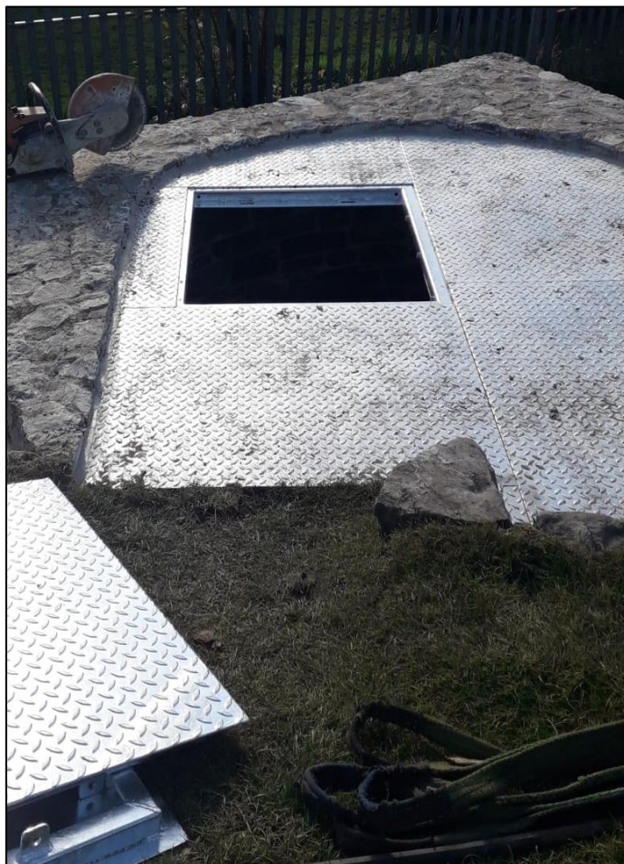
Plate 13 Roof access metal plate and trap door hatch, facing northwest
