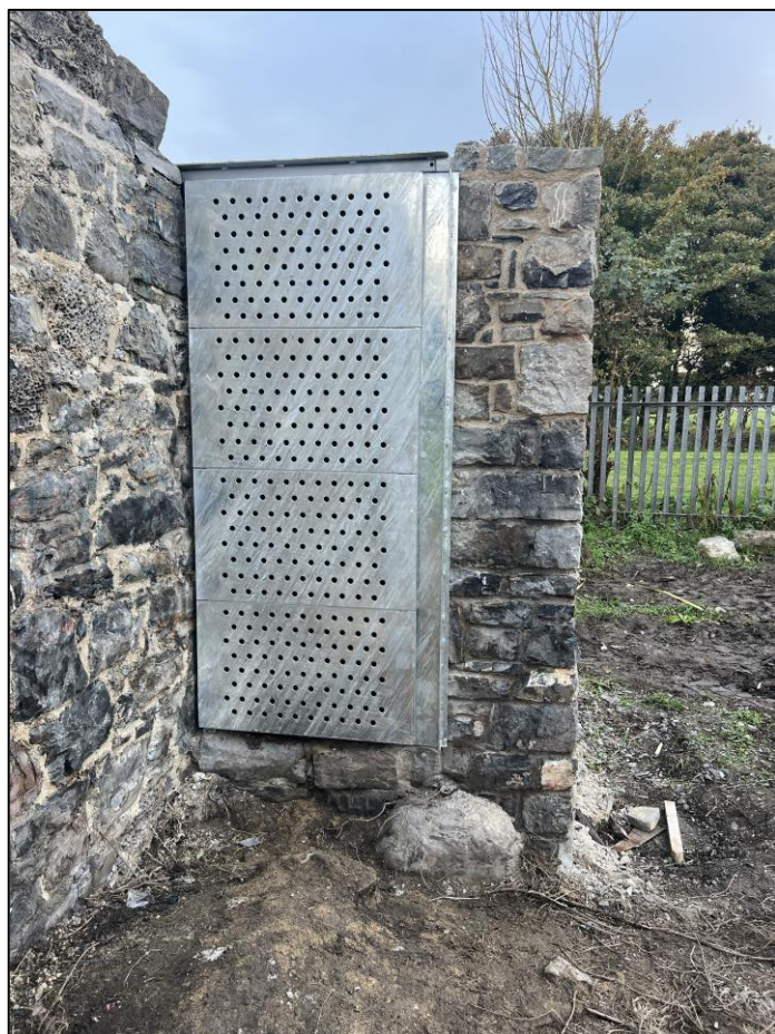
Plate 12 New steel security door on staircase/tower entrance
