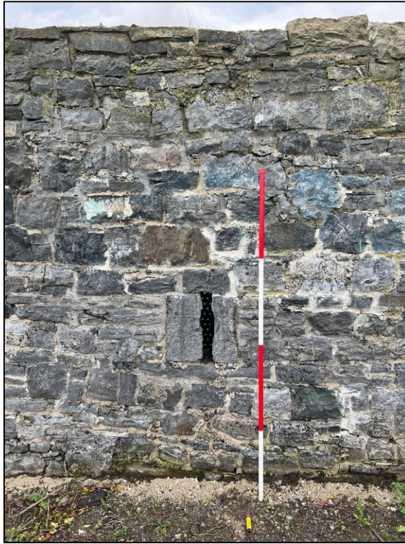
Plate 5 Eastern elevation showing height of window vs present ground level
