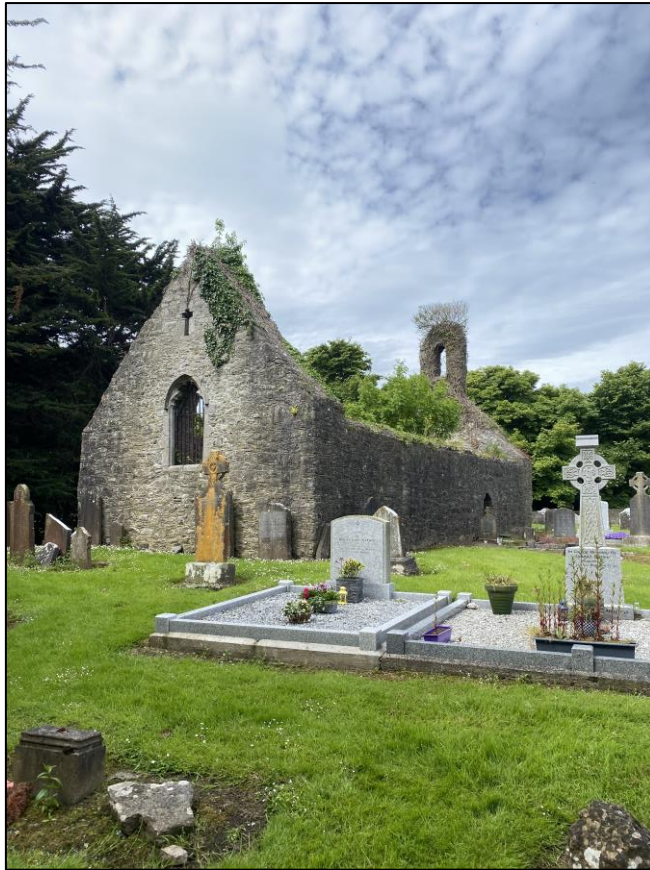
Plate 9 Exterior of eastern gable pre-commencement, with ivy in masonry crack, facing southwest
