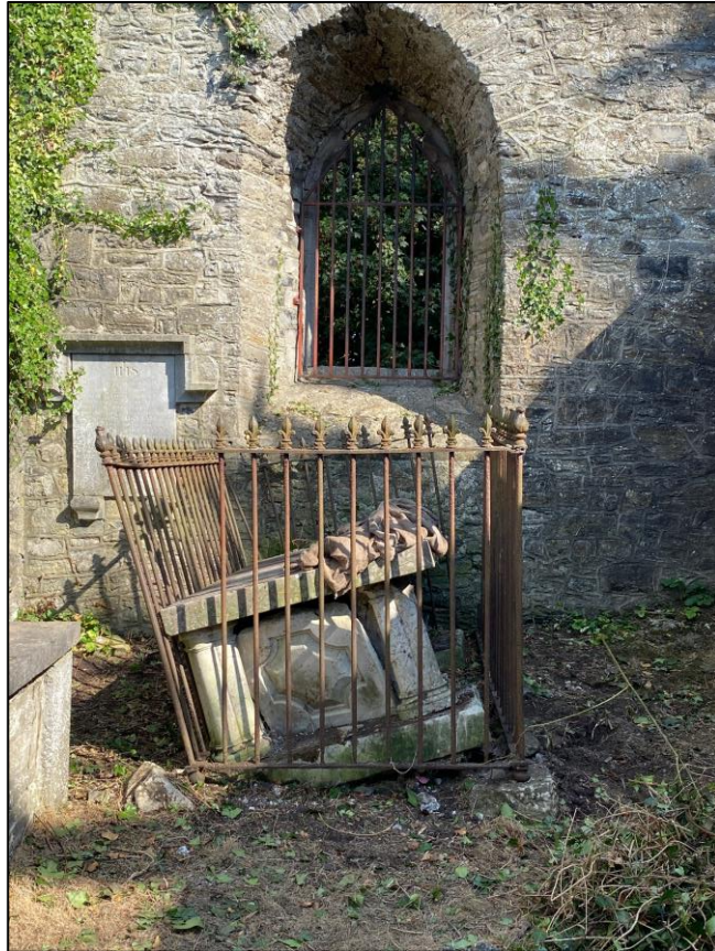
Plate 6 Subsided table tomb interior to eastern gable of church
