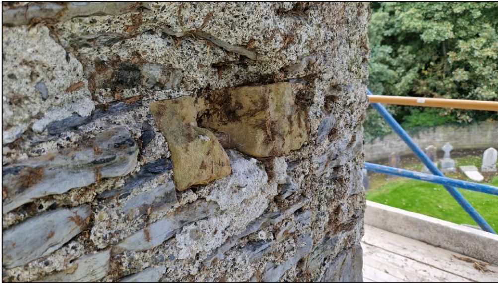
Plate 16 Yellow sandstone rebate in belltower arch, facing southwest
