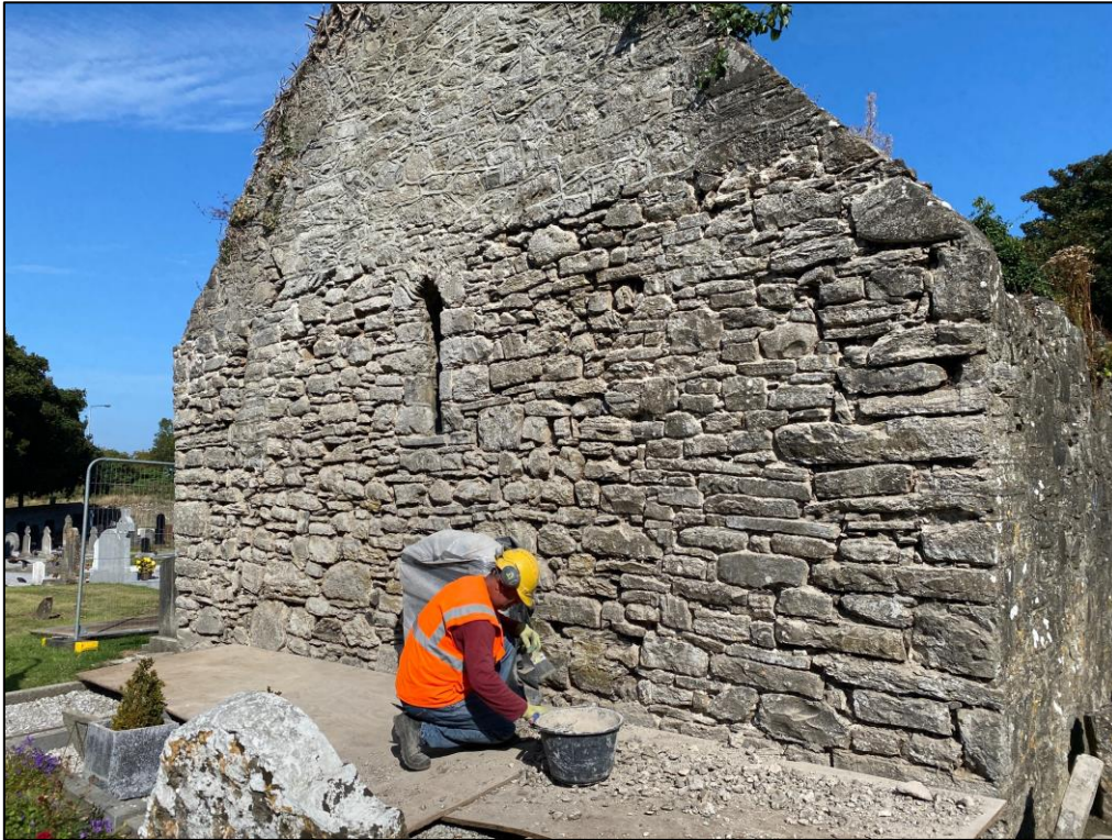
Plate 1 Removal of strap pointing exterior of western gable at ground level
