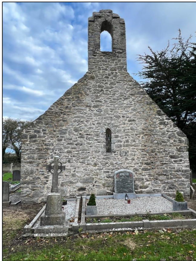
Plate 8 Exterior of western gable, post-repair and repointing
