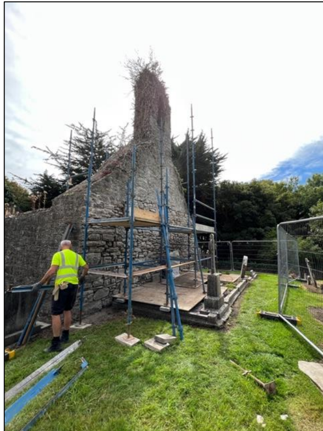
Plate 2 Scaffolding erection on western gable exterior, gravestone in bubble wrap
