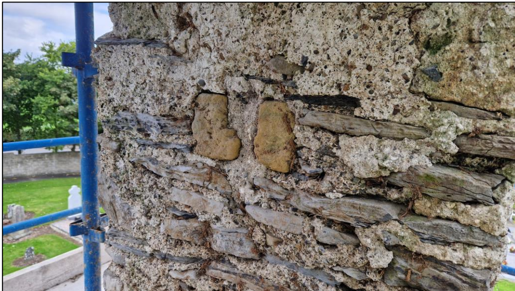
Plate 17 Yellow sandstone rebate in belltower arch, facing northeast
