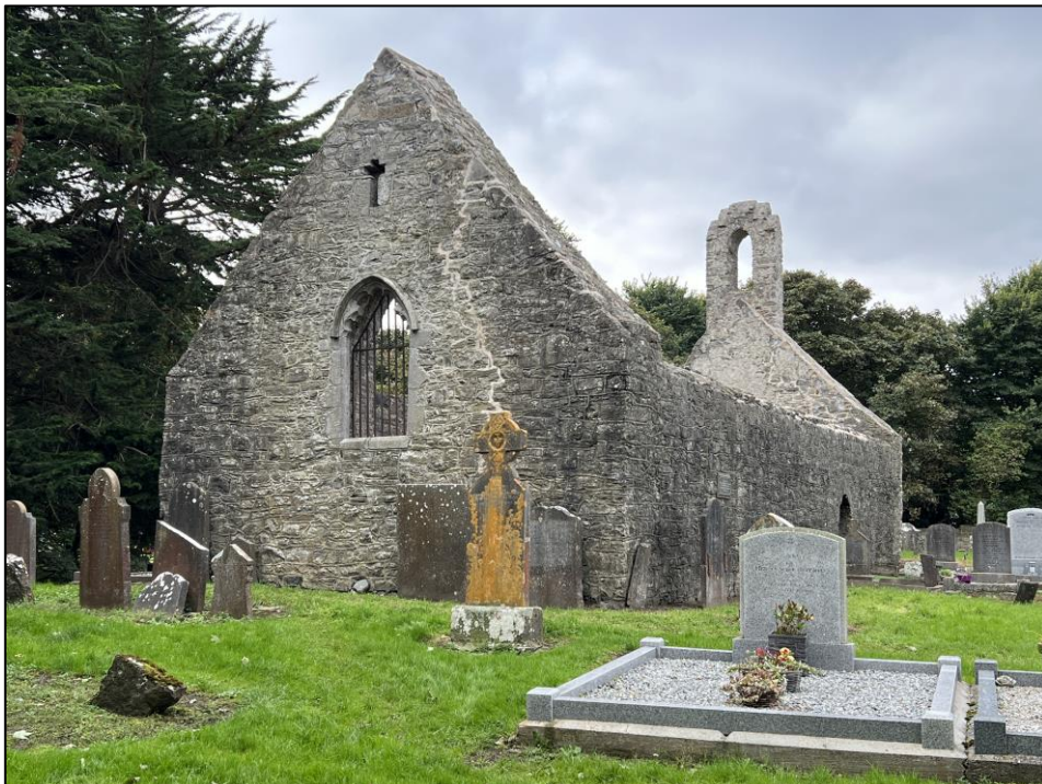
Plate 10 Exterior of eastern gable following repair, facing southwest
