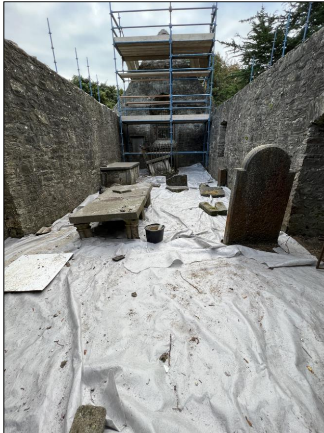
Plate11 Interior of church following geotextile imposition, facing east
