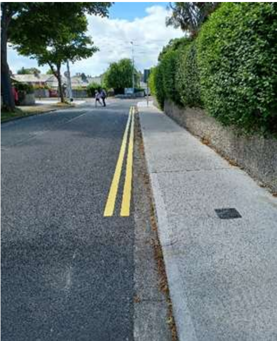
Burrowfield Road -Sutton to prevent illegal parking on the footpath
