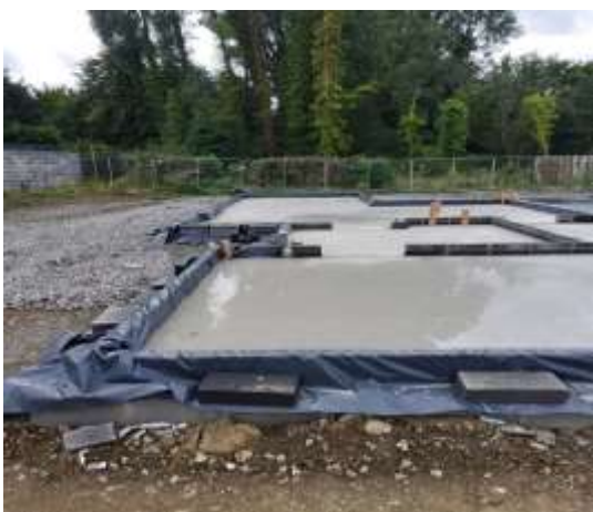
Ground floor slab freshly poured in a housing development in Castleknock.
