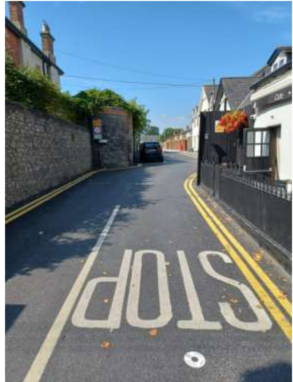
St Margaret's Road, Road Inlay
