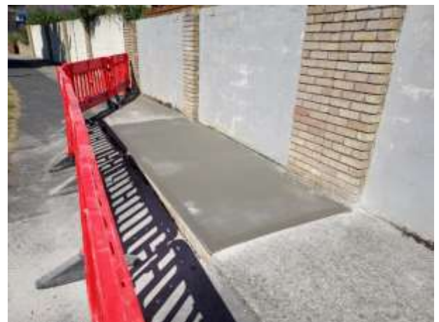
New footpath sections at Dun Emer Avenue, Lusk
