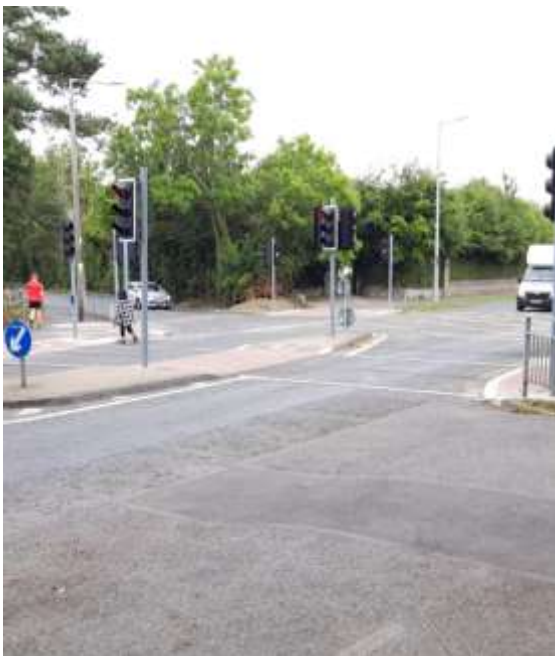
Junction upgrade at Snugborough Road and Grove Road
