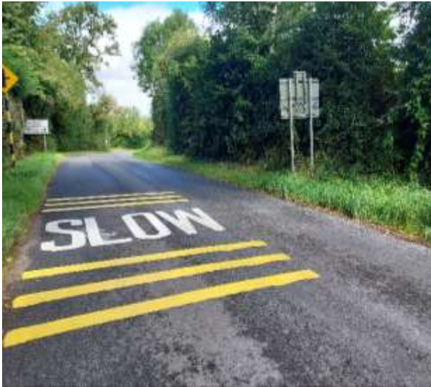
R122/R129 – New and refreshed lining on the approach of the junction
