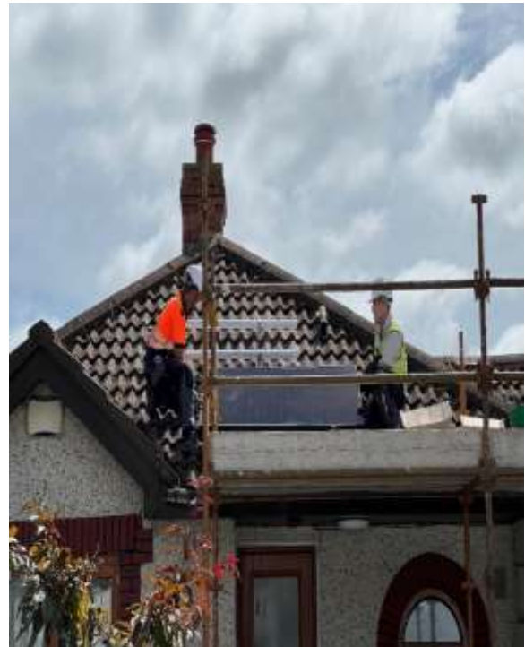
PV panel installation in Jugback Estate
