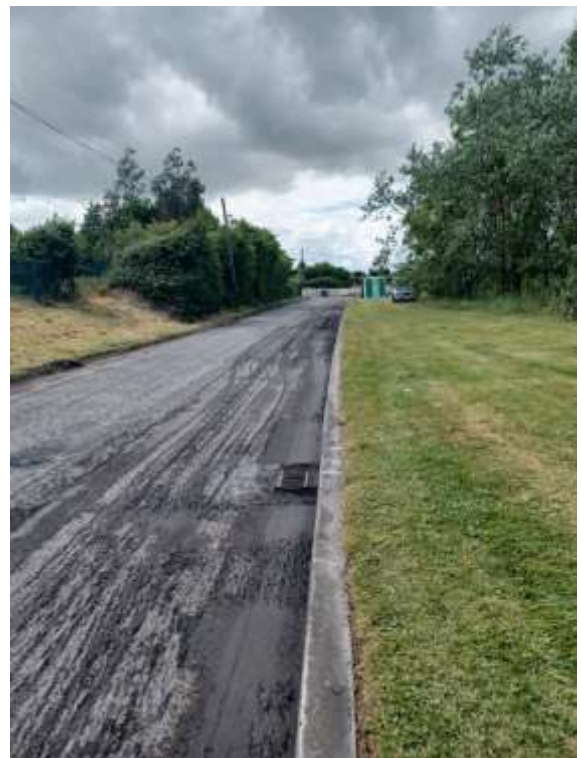
Estuary Road, Road Inlay
