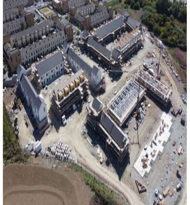
Fingal County Council construction scheme at Church Fields - 67 units being built
