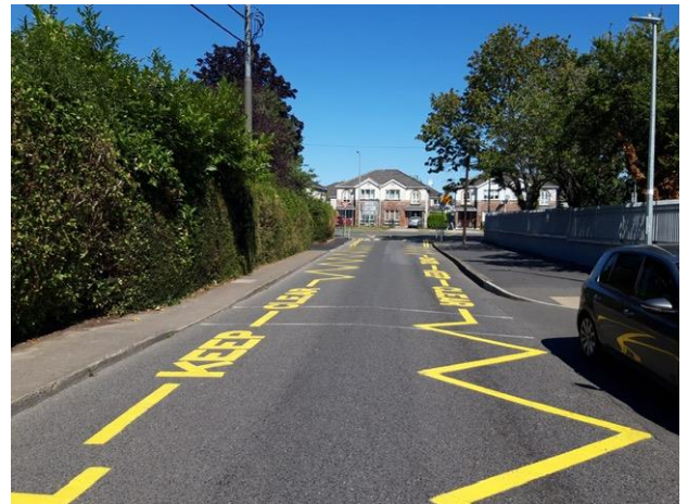
The road lining was refreshed outside St. Mochta's National School on both the Porterstown Road and the Clonsilla Road
