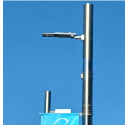
Testing of Balbriggan main streets new LED system under way
