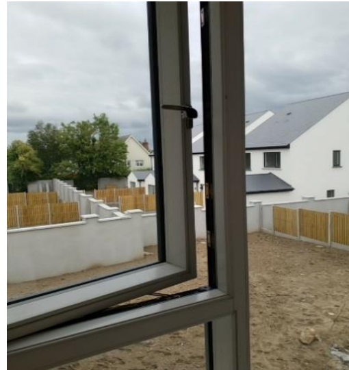
Checking a window opening restrictor in a house in Rolestown
