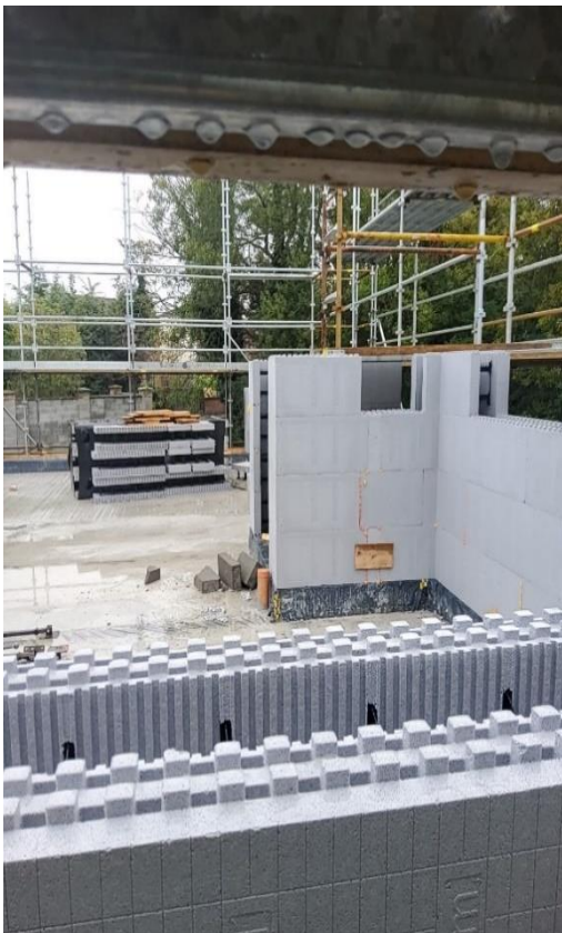
An Insulated concrete formwork (ICF) house under construction in Castleknock
