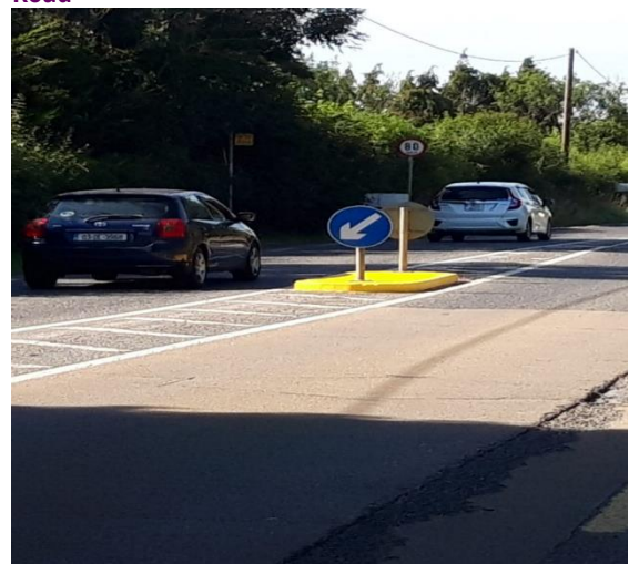
The central island on the R135 at Coolquay Gateway has been fully painted yellow to endorse visibility of the island when approaching the gateway
