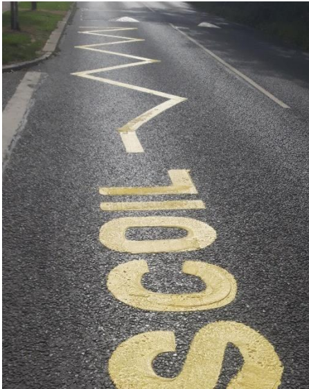
Donabate - Beaverstown Road @ Educate Together - Traffic Calming Ramps & School Lining
