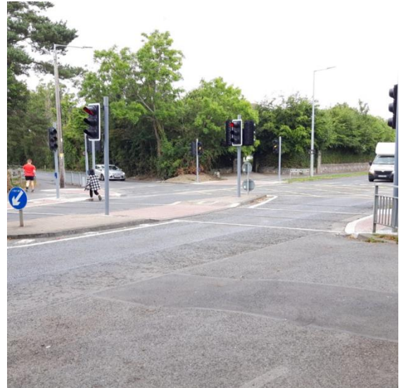
Junction upgrade at Snugborough Road and Grove Road
