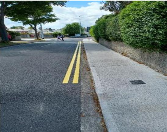
Burrowfield Road, Sutton to prevent illegal parking on the footpath
