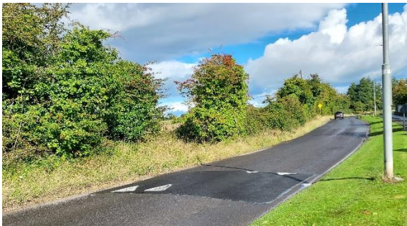
Lusk- New Traffic Calming Ramps at Minister's Road works in progress
