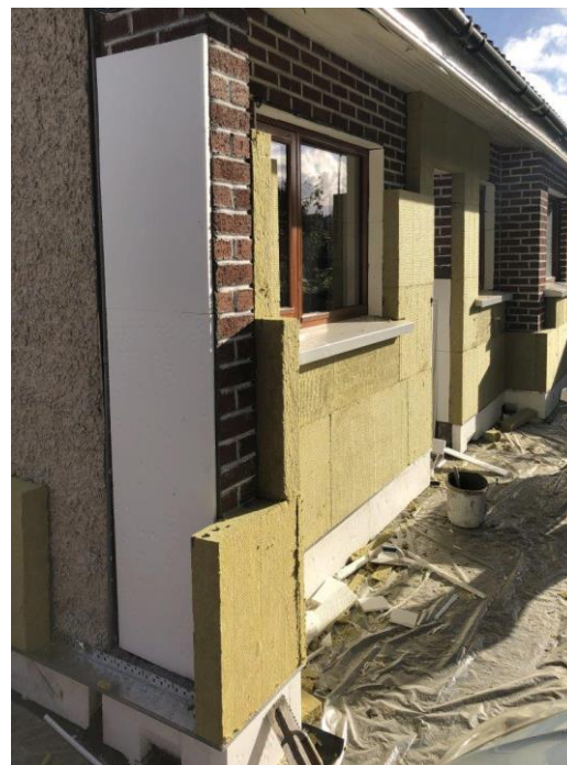
External wall insulation being installed as part of extensive retrofit upgrade
