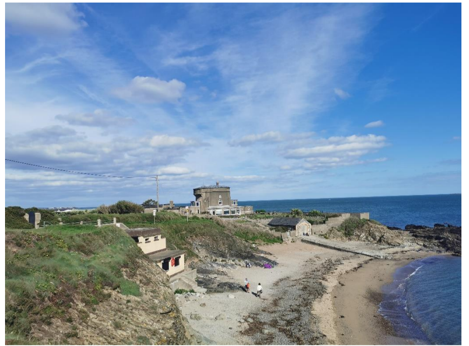
Plate 65: Quay 14.4 Martello Tower (DU012-010-) from S
