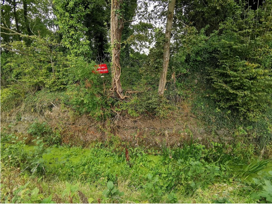
Plate 11: Bridge at Tide Mill 2.4 from E
