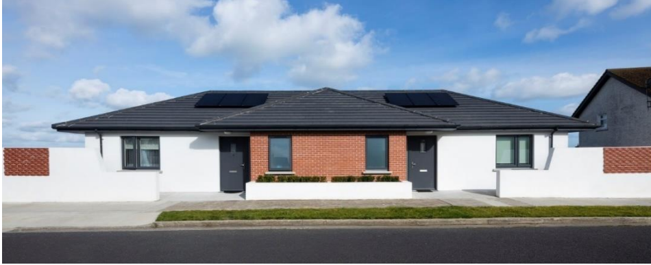
Pinewood Housing Estate, Balbriggan. Completed in 2021, all units have a BER rating of A2 and achieved NZEB standards.
