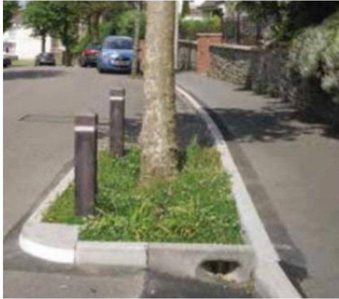
An example of an integrated constructed tree pit which can be installed to absorb surface water runoff.
