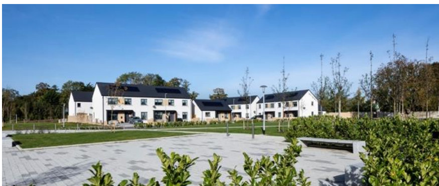
Rowlestown Estate. Completed in 2021, all units have a BER rating of A2 and achieved NZEB standards
