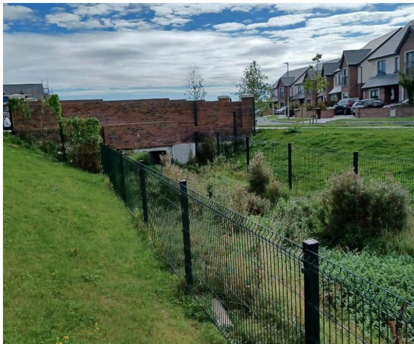
An example of a natural watercourse that was retained, through a new residential development, which allows for attenuate water to be discharge into.
