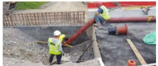
Ductile Iron foul rising main being laid across the bridge
