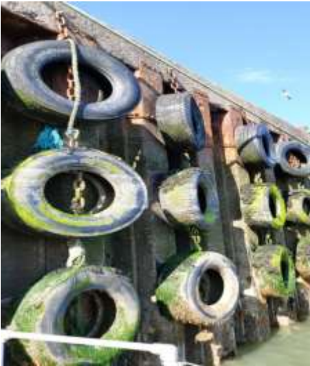
Figure Tyre and chain fenders at Skerries Pier
