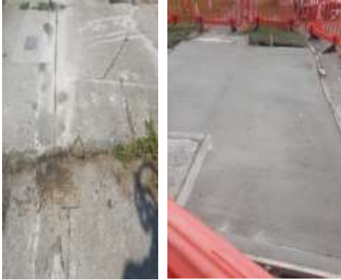
Concrete Repairs St Cronan's Close Swords
