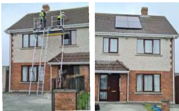
Pre and Post Energy Efficiency Retrofitting Works – Solar Panels
