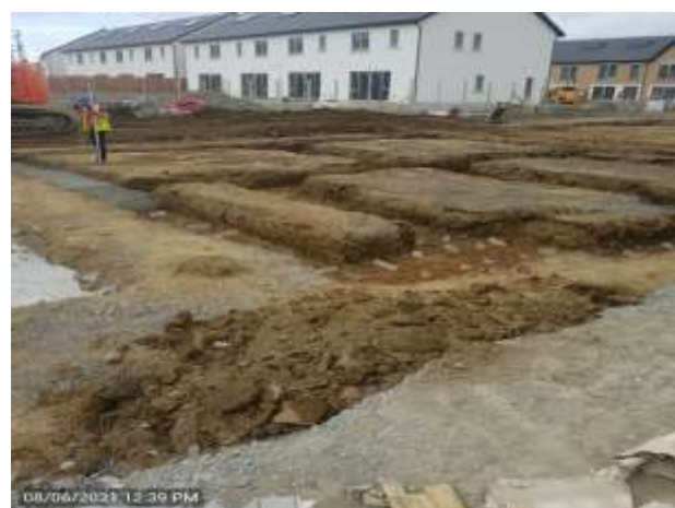
June 2021 – Foundation for houses in the Hollywoodrath development being poured.
