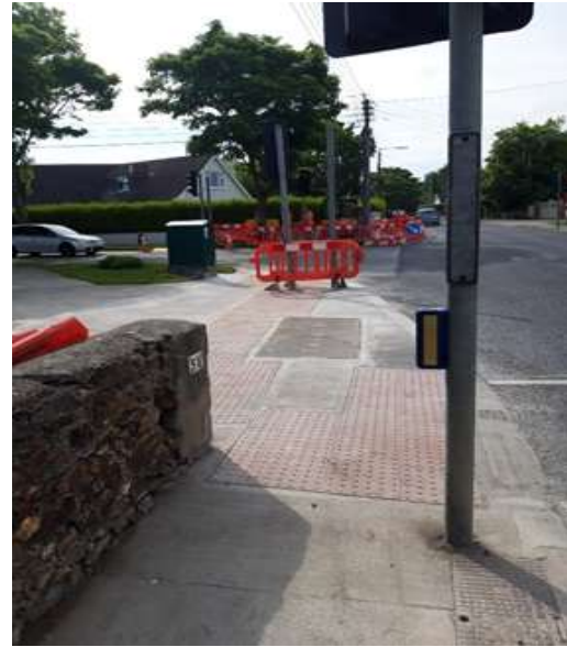
Upgrade of Pedestrian Crossings at Carrickbrack Road - Offington Park Road junction
