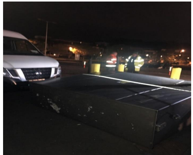
ESB sub-station overturned from impact of car accident.
