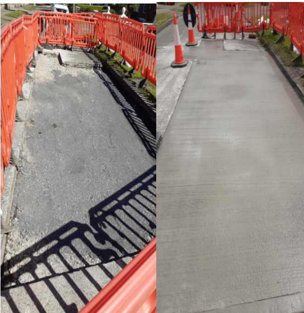
Concrete Repairs Santry Close
