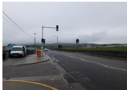
New Traffic Signals on Greenfields Road - Sutton now in operation
