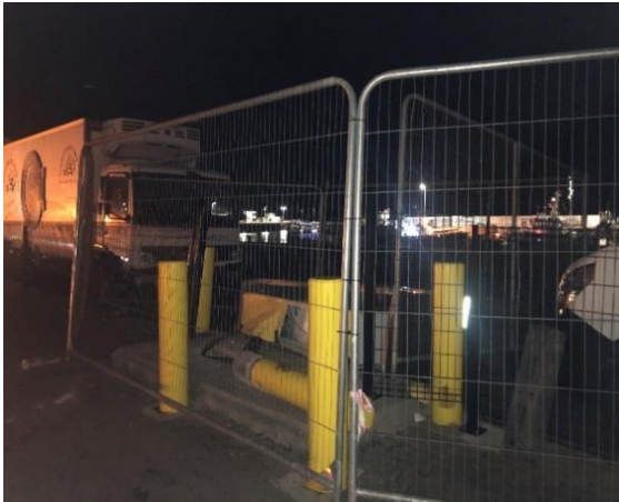
Heras fencing erected by On Call Crew leaving ESB sub-station safe
