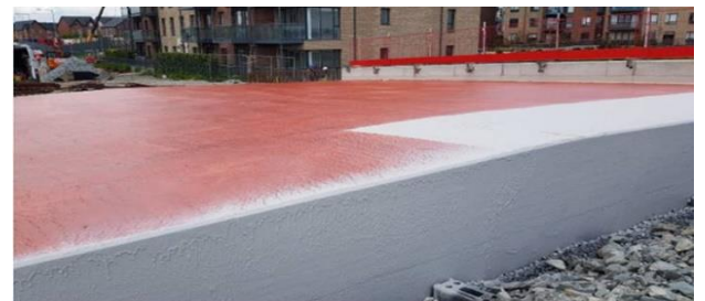
Bridge Deck poured, cured and waterproofed
