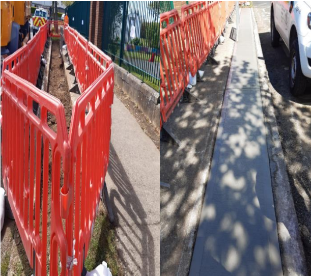
Concrete Repairs Rivermeade
