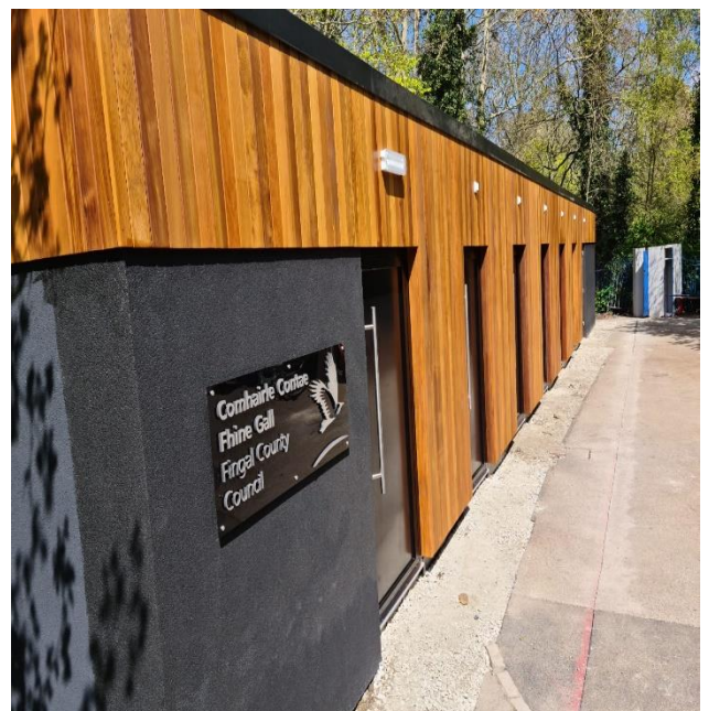
Construction almost complete of replacement toilets at Newbridge Demesne Playground
