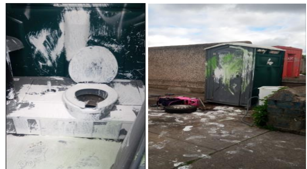
Damage to Portable Toilets - St Mary’s
