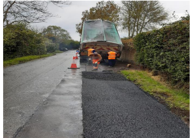
Road Patching at Balheary Road
