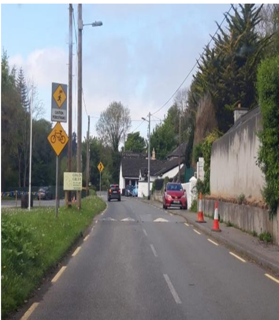
Cyclist Warning signs erected along the length of Lower Road
