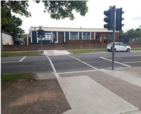
Tactile paving upgraded on Feltrim road by Scoil an Duinnígh. The foreground tactile paving is completely new as a previous tree (now removed) prevented tactile being present because of tree roots.
