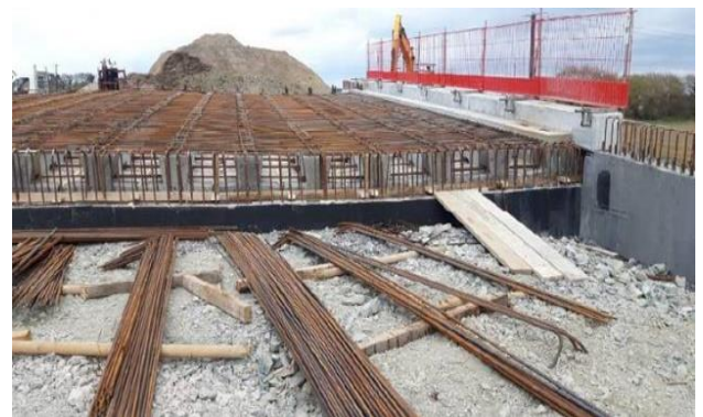
Steel fixing for bridge deck
