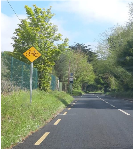
Cyclist Warning signs erected along the length of Lower Road
