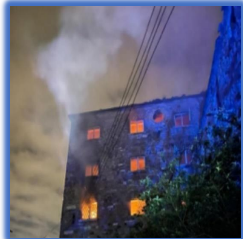
Fire in Ashtown Mill – structure and place assessed by BC Engineer
