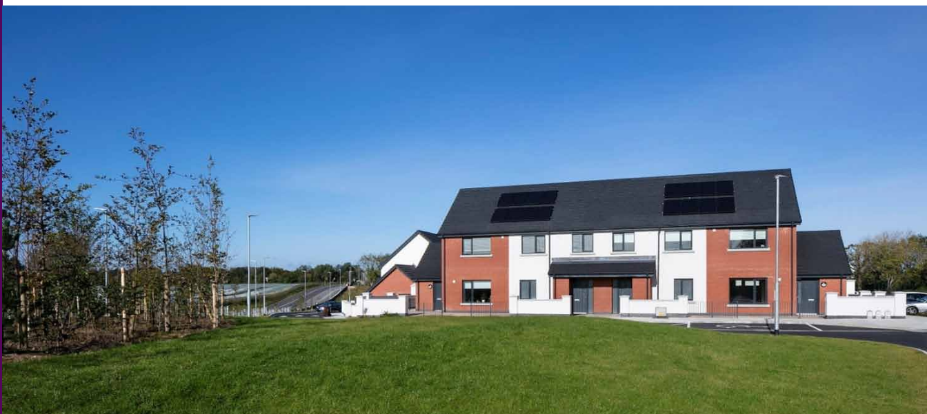
Holymount Estate, Rathbeale Road, Swords. Completed in 2020, all 24 units have a BER rating of A2 and achieved NZEB standards
