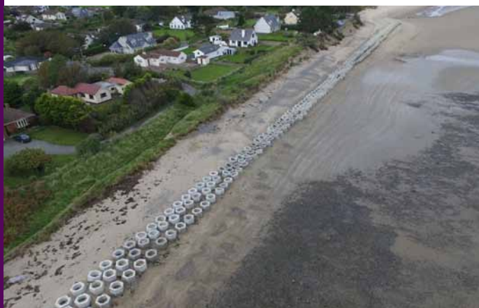
Seabee concrete units on the Burrow Beach in Portrane
