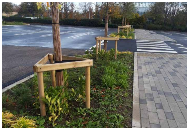
Tree pits at Blanchardstown Shopping centre, an example of provision of SuDS through the planning process
