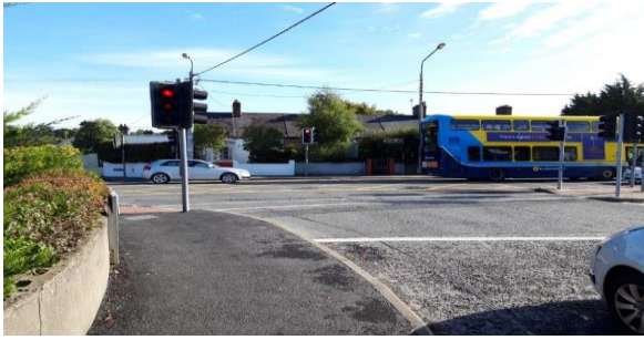
Footpath widened at Blanchardstown Main Street/Clonsilla Road junction
