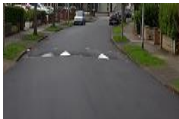
Newly installed Ramp - The Avenue, Rush, at St Catherine's National School
