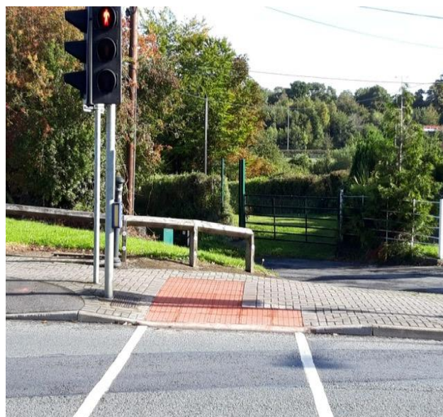
New tactile paving installed at Blanchardstown Main Street/Clonsilla Road junction
