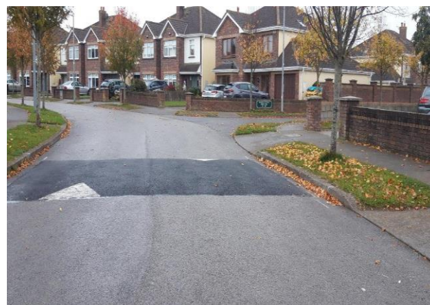
Newly installed Ramp - Carr's Mill, Donabate
