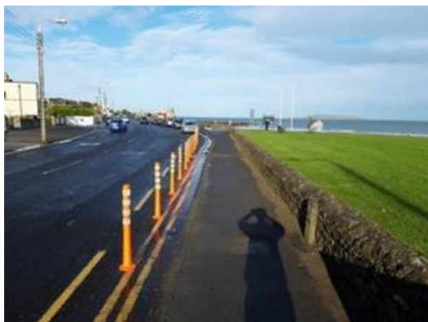
New Bollards - Coast road Portmarnock
