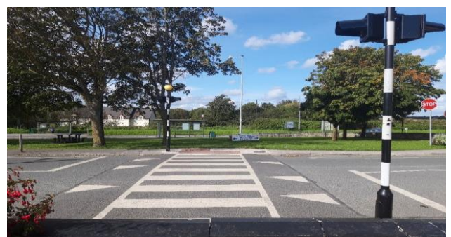
Balrothery Village - New Zebra Crossing was commissioned in October.
