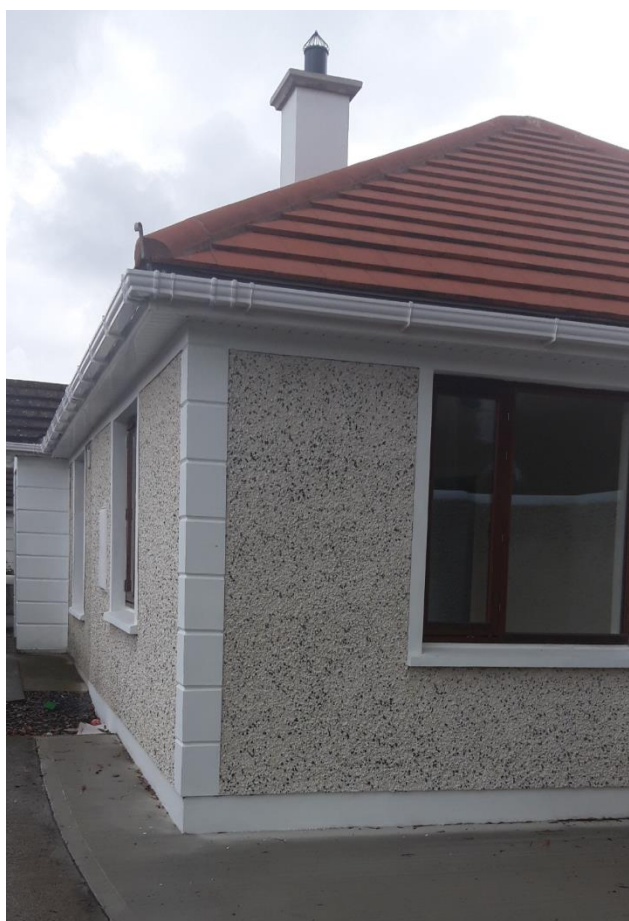
Newly built extension at Traveller Specific Group Housing Scheme Meakstown Close
