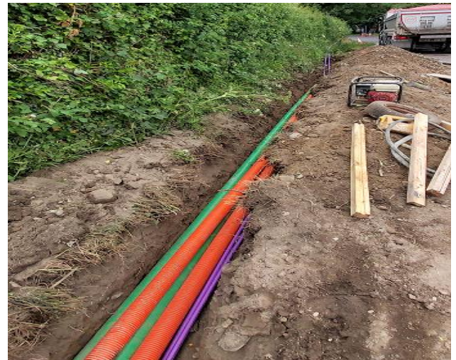
Ducting installation in Roganstown Co. Dublin.
