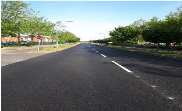
Resurfacing of Castlecurragh Road
