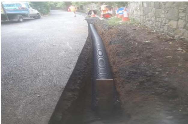
Drainage Works – Somerton Lane
