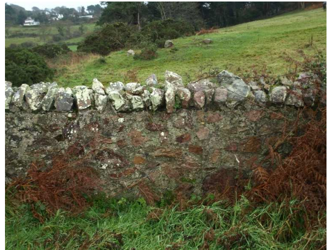
Figure 18: existing stone wall
