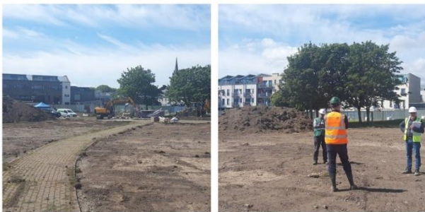
Works progressing on Village Green, Malahide
