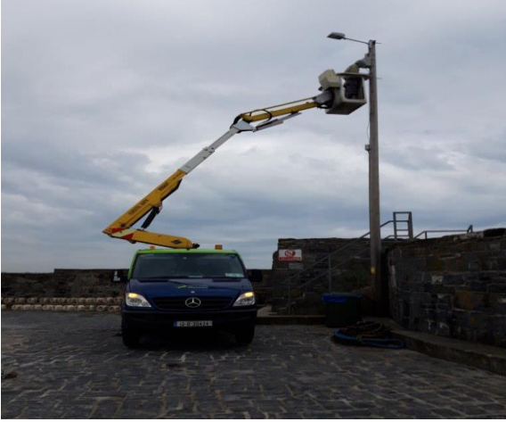
Repairs carried out at Rush Harbour
