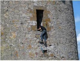
Figure 30: Martello tower showing door opening and missing brickwork
