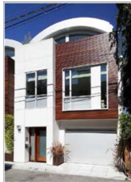
Figure 5.41 Well designed integrated garages can reduce the requirement for on-street car parking.
