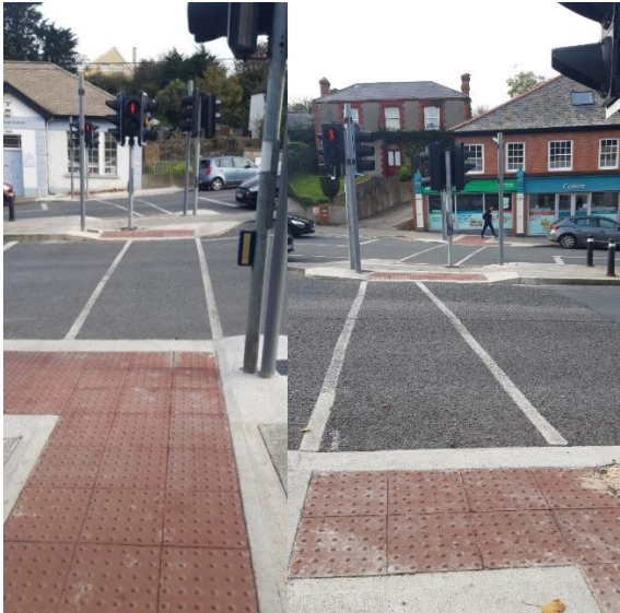
Main Street Howth: New crossing from both sides with new tactiles and wider tram lines
