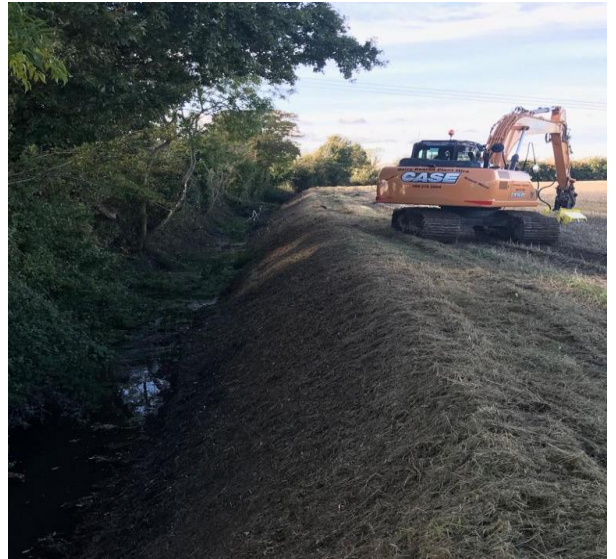
Section of stream after works completed
