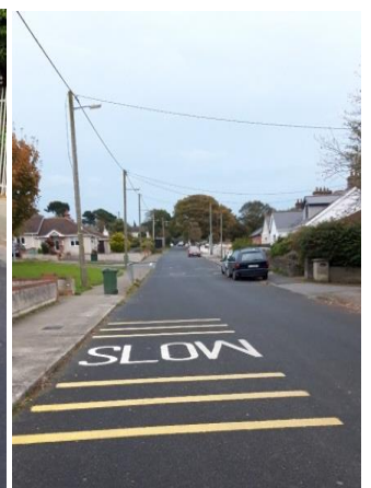
Road markings recently installed in Seamount, Malahide
