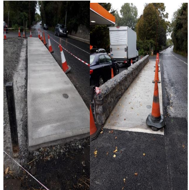
New stone wall and footpath in Hollystown
