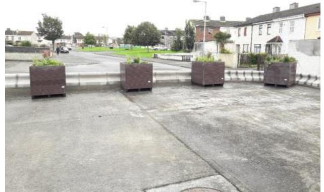
Planters installed in Fortlawn Estate
