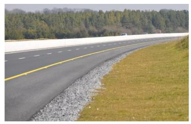
Figure 6.7 Example Filter Drain
