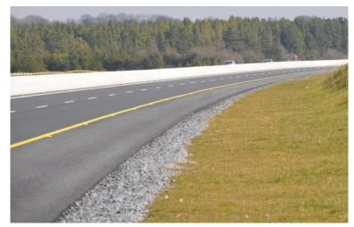
Figure 6.7 Example Filter Drain
