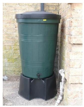
Figure 6.2 Domestic Water Butt (Susdrain.org)
