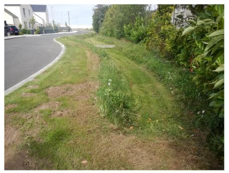
Figure 6.10 Example Roadside Swale
