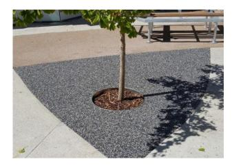
Photo 3.6.3 Tree Pit (Source: www.waterpave.com.au)
