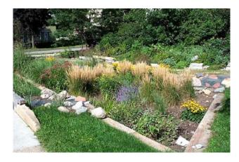
Photo 3.7.2 Bioretention Area/ Rain Garden (source: www.designingbuildings.co.uk)
