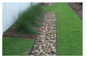
Photo 3.6.7 Infiltration trenches/ soakaways (source; www.sudswales.com)
