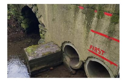
Photo 2.3.1 Three culverts under the road at western boundary
