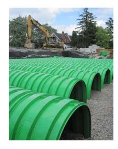
Photo 3.7.4 A Triton<sup>™</sup> Subsurface Attenuation System (source: www. http://terrafixgeo.com )
