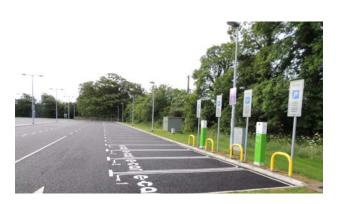
Photo 3.6.4 Example of a Porous Ssphaltic Surface (Duraflow ® System) at Luas Park and Ride (Source www.roadstone.ie )
