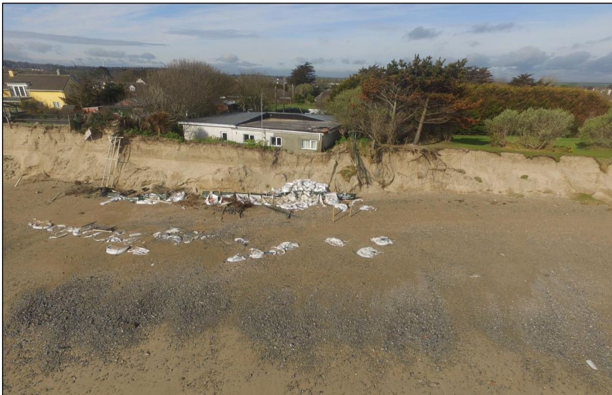
Figure 4.1: Residential property D is now perched on the edge an over-steepened dune.
