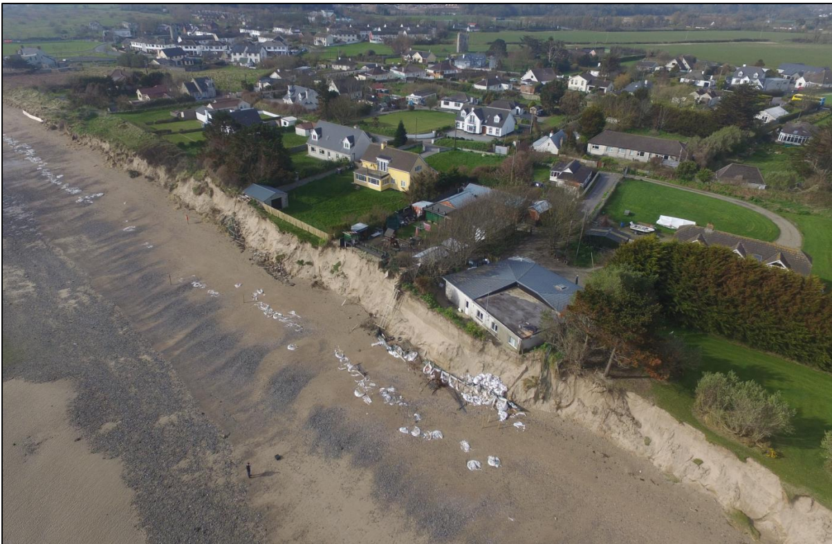
Figure 4.5: Aerial view of the threatened residential properties along the southern section of the Burrow.
