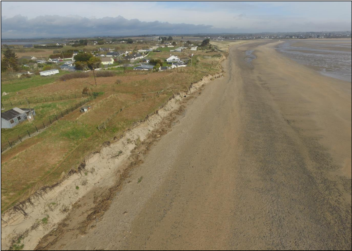
Figure 4.4 Extent and magnitude of dune erosion along the mid-section of the Burrow – looking north.
