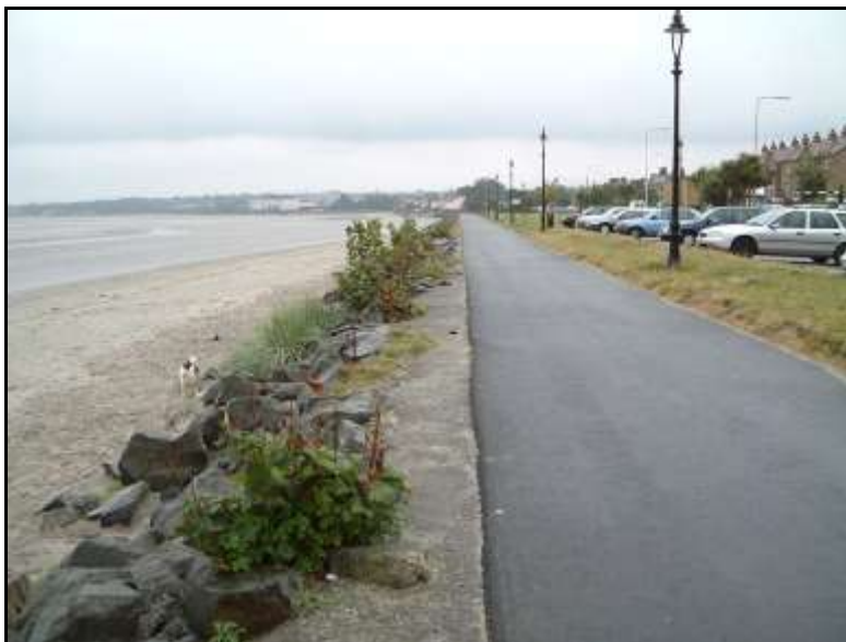
Figure 18.19 - Sandymount Strand Promenade Looking South
