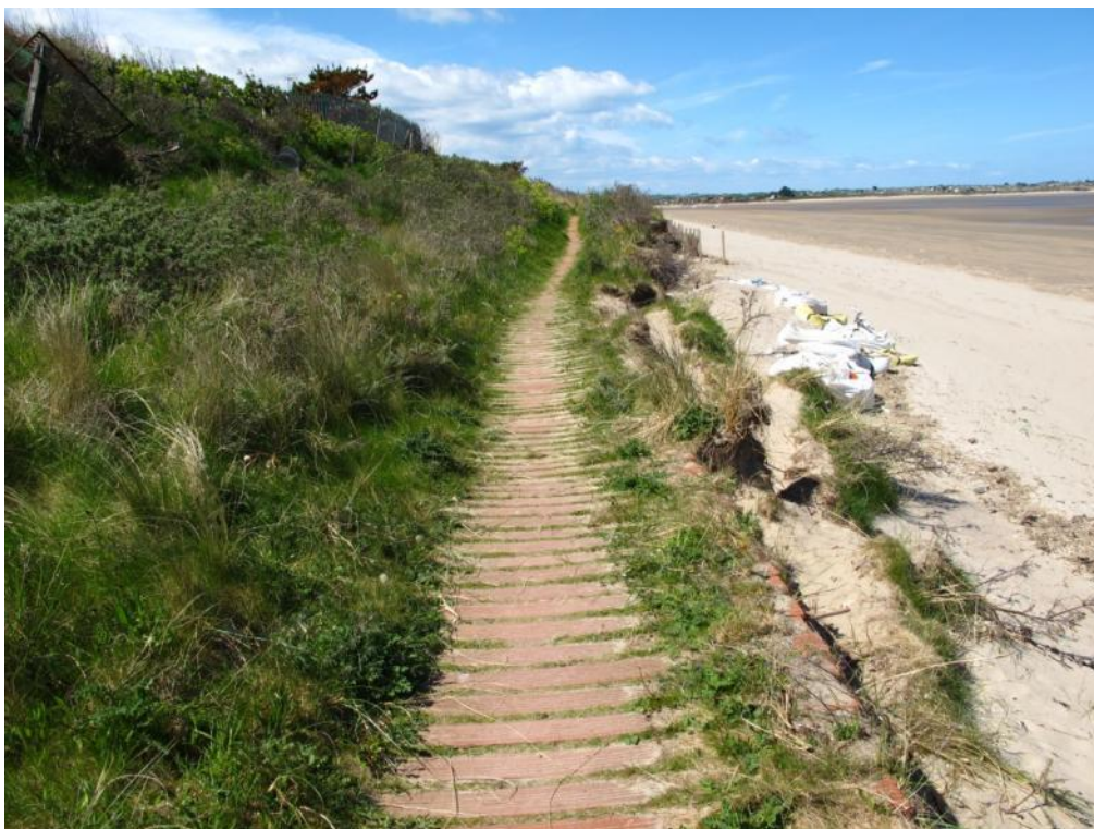
Figure 5.1.6: Wooden boardwalk with erosion damage, south end of beach (looking north)
