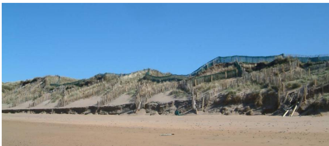
Figure 12.7.2: Sand trap fencing damage following typical winter storm event Co. Clare
