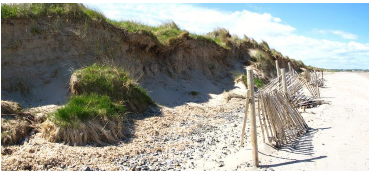
Figure 5.1.5: Erosion damage, southern end of beach (looking north)
