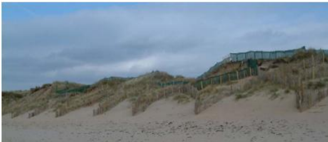
Figure 12.7.1: Sand trap fencing being employed successfully at Co. Clare
