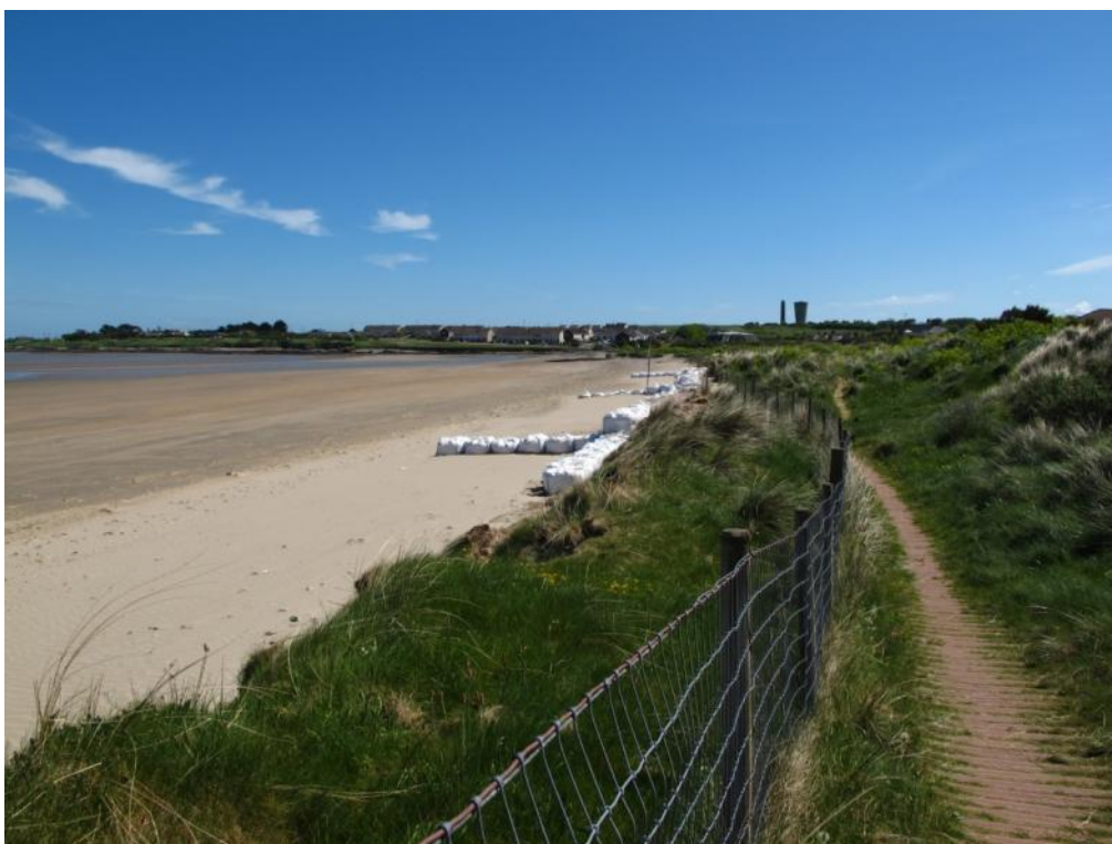
Figure 5.1.7: Wooden boardwalk view south showing erosion protection sandbags
