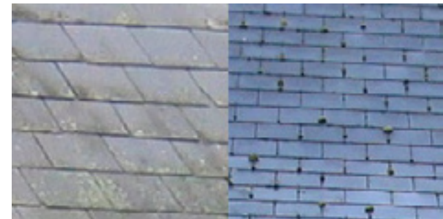
Fig. 4.1.2 Examples of existing Natural Slate roofs in Garristown
