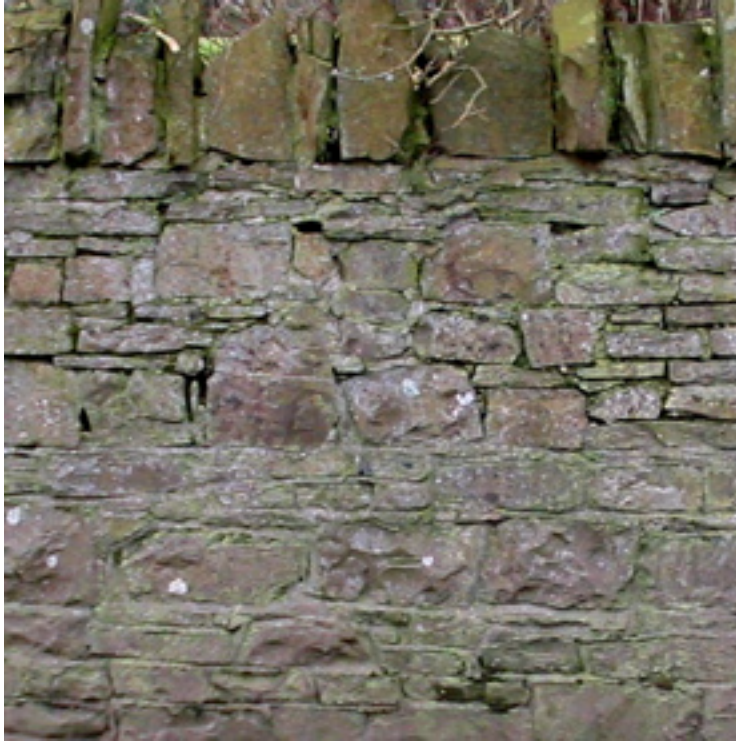
Fig. 4.2.6a Existing retaining wall facing the Naul Road.
