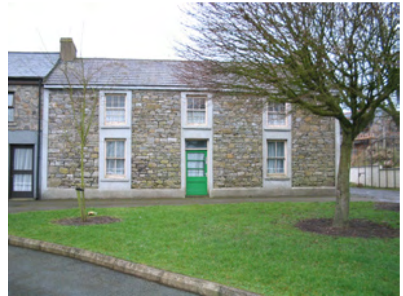
Fig. 4.1.1 Existing building on Main St
