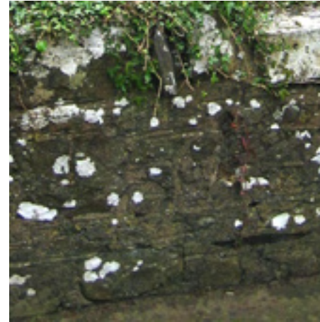
Fig. 4.2.6b Existing wall around the cemetery
