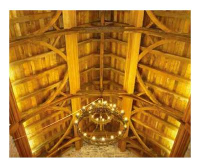
PLATES 20 AND 21: Interior of Chapel, east end, showing tiled floor (based on historic pavement) and the timber roof
