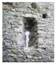
**PLATE 42:** 'Keyhole' ope at first-floor, south wall of East Tower
