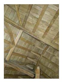
PLATE 58: Constable's Tower interior, top floor. View of new roof trusses and boarding
