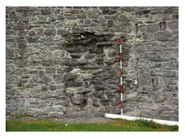
PLATE 46: Restored wall showing original fabric
