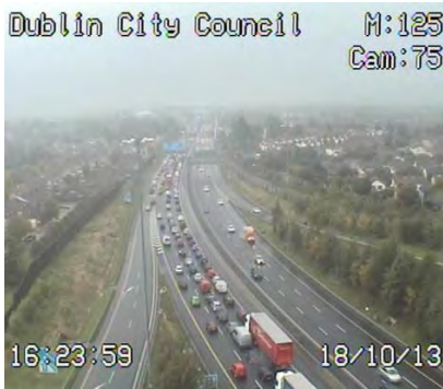
Photo 2.1 – M50 Firhouse – PM
