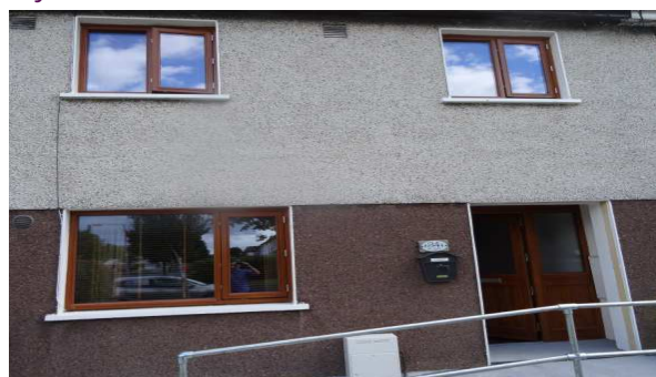
Example of Window & Door Replacement in Dublin 15
