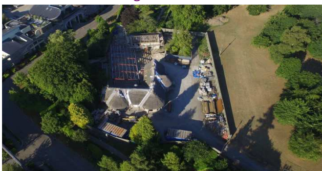
Aerial view of the on-going works at the Casino
