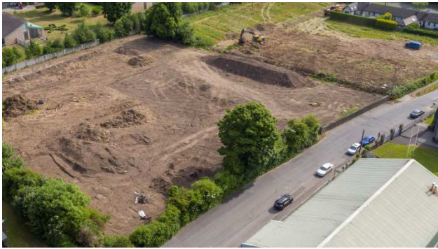
Work has commenced on the Rowlestown site
