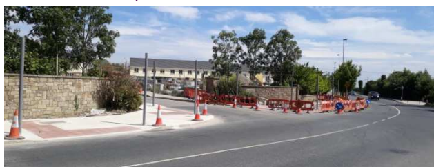
Cappagh/Heathfield traffic signal junction under construction
