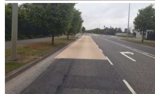
Cruisath Road, Damestown
