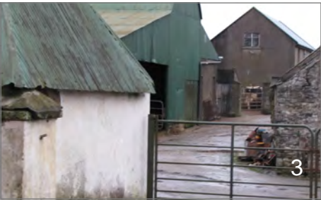
3 and 4: Farm outbuildings at southern end of village (west side). The roadside building appears to be a mud structure with previously thatched roof. Stone gable buildings also appear to have architectural merit.
