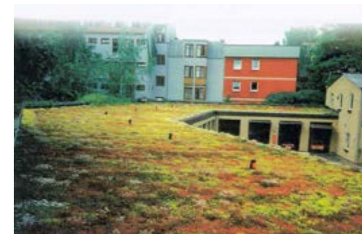
Figure A.19 Extensive Greenroof system
