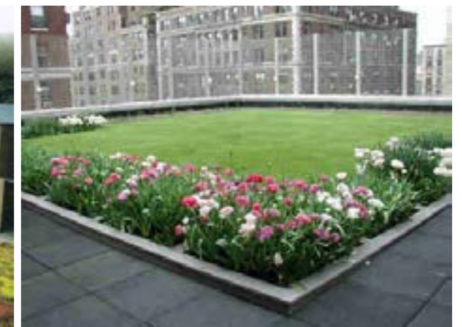
Figure A.20 Intensive Greenroof system
