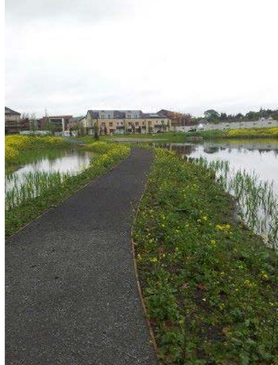
Figure A.8 Stormwater Wetland
