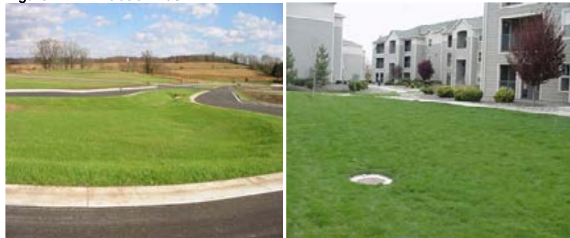
Figure A.11 Infiltration Basin
