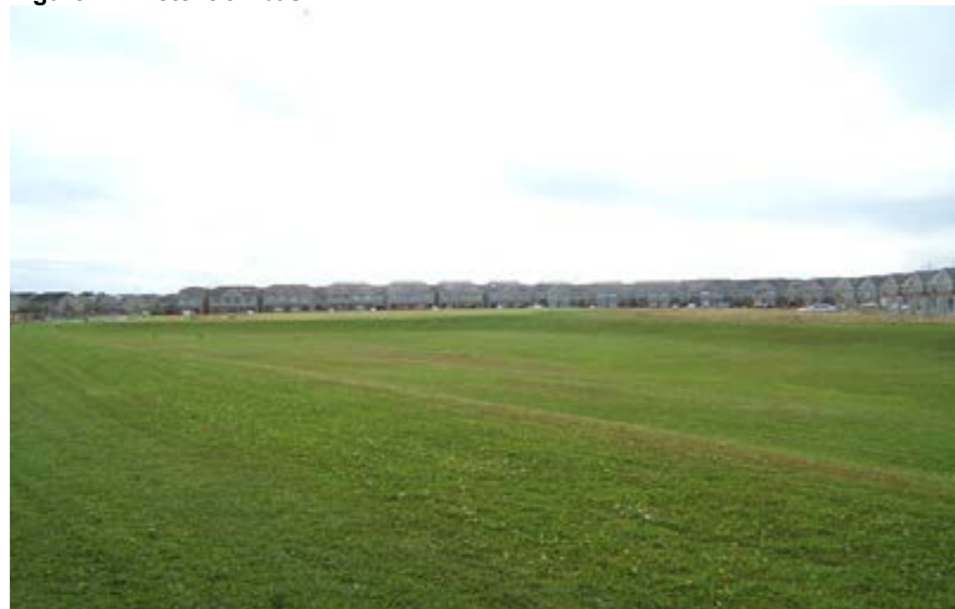
Figure A.4 Detention basin
