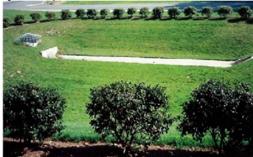
Figure A.3 Example of a Detention basin
