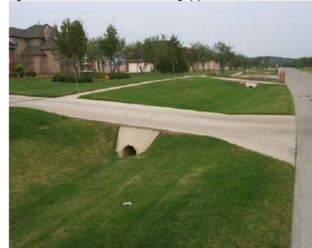
Figure A.15 Swale – Flow restriction through pipe diameter
